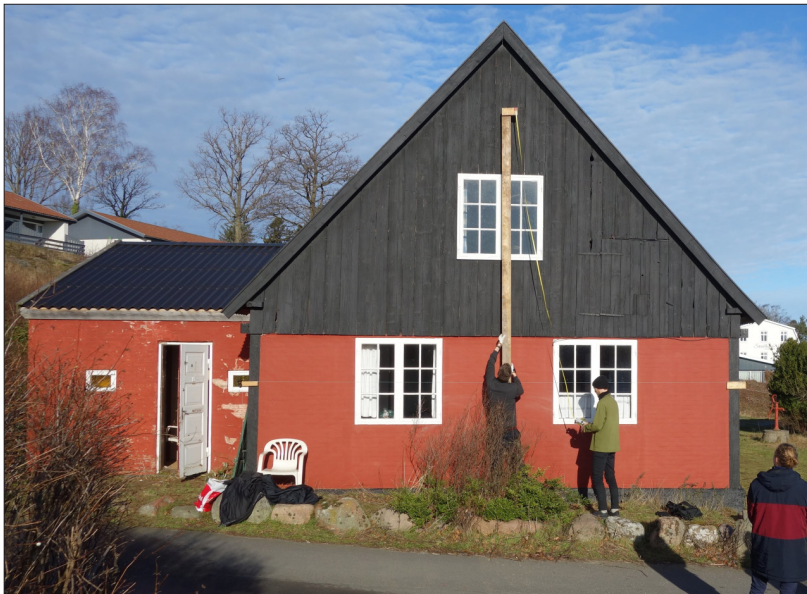
Figure 1. 'The Apprentices' House' as it looked when the project started in 2018 with a raised Eternit slate roof, plastic-painted walls, plinth, and half-timbering. Photo: Thomas Kampmann.
