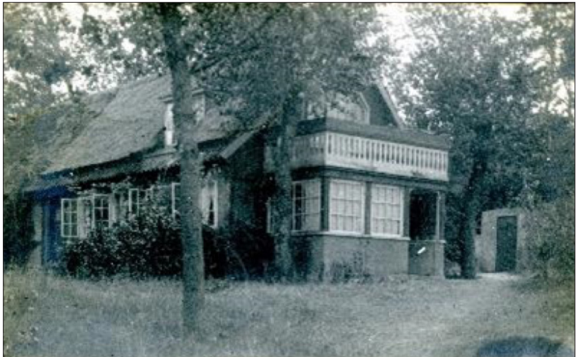
Figure A.7. Historical picture of the house viewed from the north. Private photo from Martin Silbersteins archive on Bornholms Ø-arkiv, BØA 1980-20-2.
