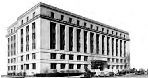
Figure 2. Envelope condition prior to retrofitting
