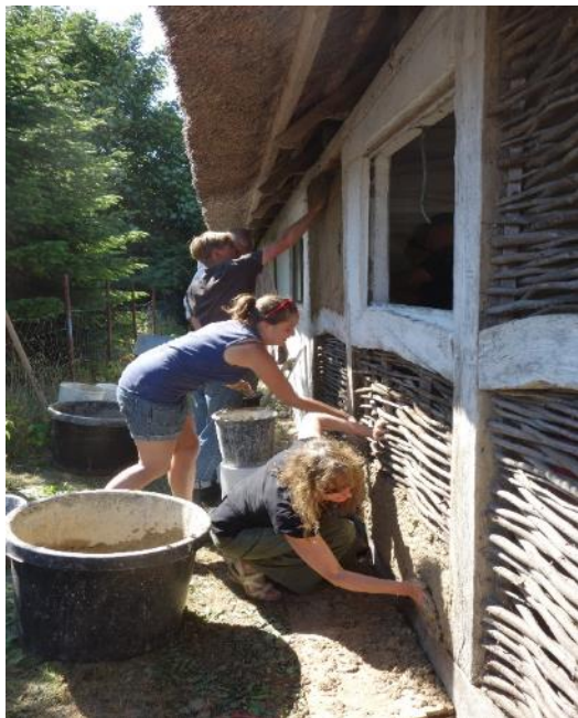
Figure 3. The execution of the wattle and daub in 2013.
