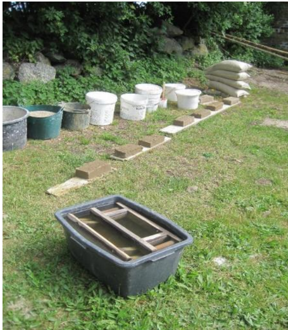
Figure 4. The wooden forms and the sundried clay stones to the adobe fillings. Photo: Søren Vadstrup.
