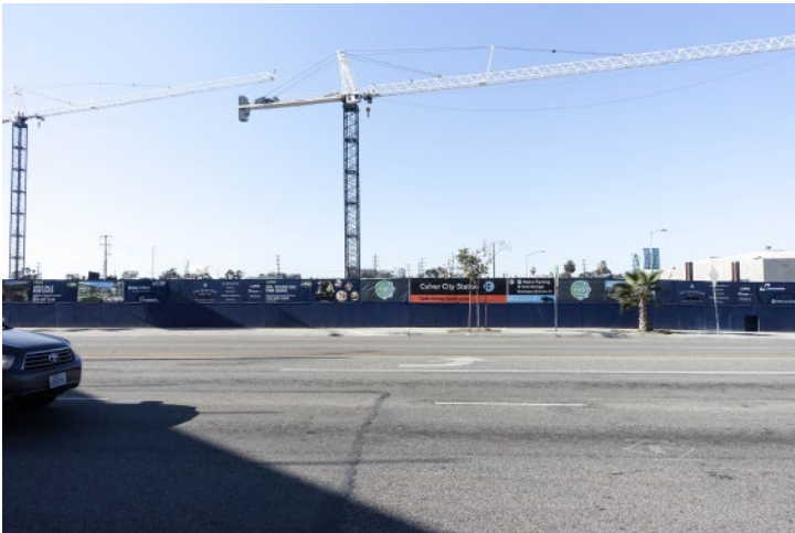
Figure 5. The future Culver City Station of Los Angeles Expo Line
