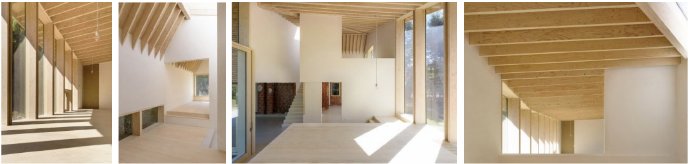
Fig. 14-17. Interior photograph of the built roof structure
