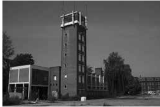
A former fire brigade station in Maastricht – before renovation and repurposing
