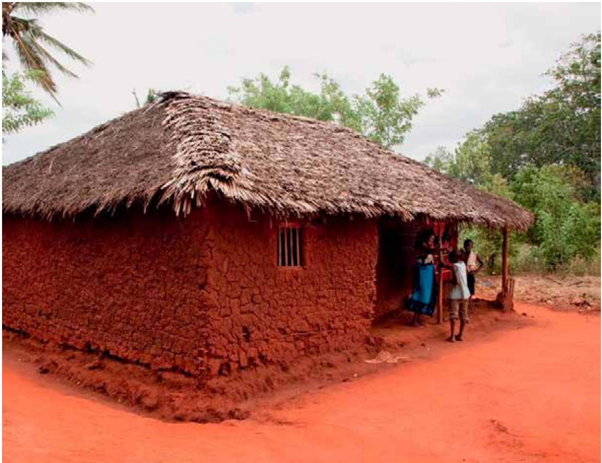
Figure 1: Typical traditional rural house in Magoda, Tanzania: a wattle and daub construction or mud house.
