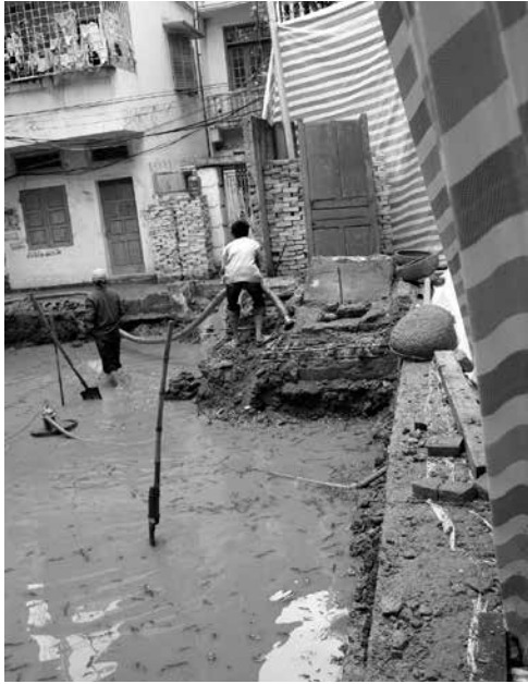
FIGURE 6 Septic tank emptying
