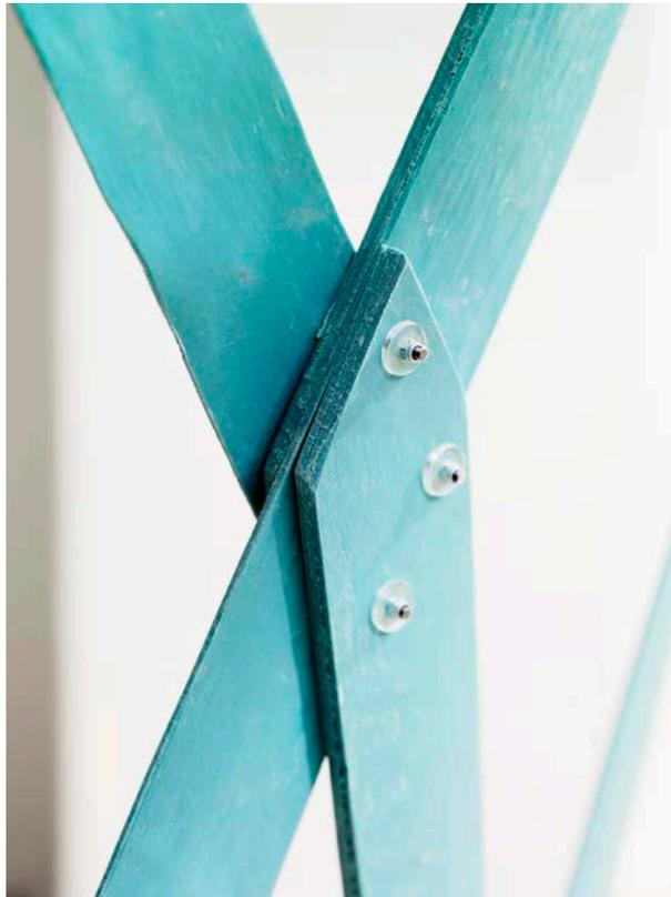
Figure 7: Stiff joints are attained through overlay and afford easy assembly
