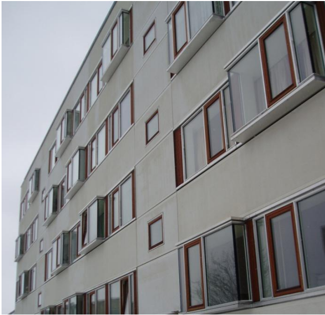
Gyldenrisparken built in 1964 Architects, renovation: Witraz, Vandkunsten 2005-10
