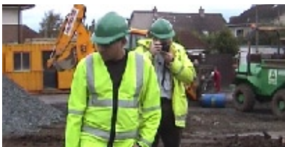
Figure 2: ... inspecting and documenting work in progress
