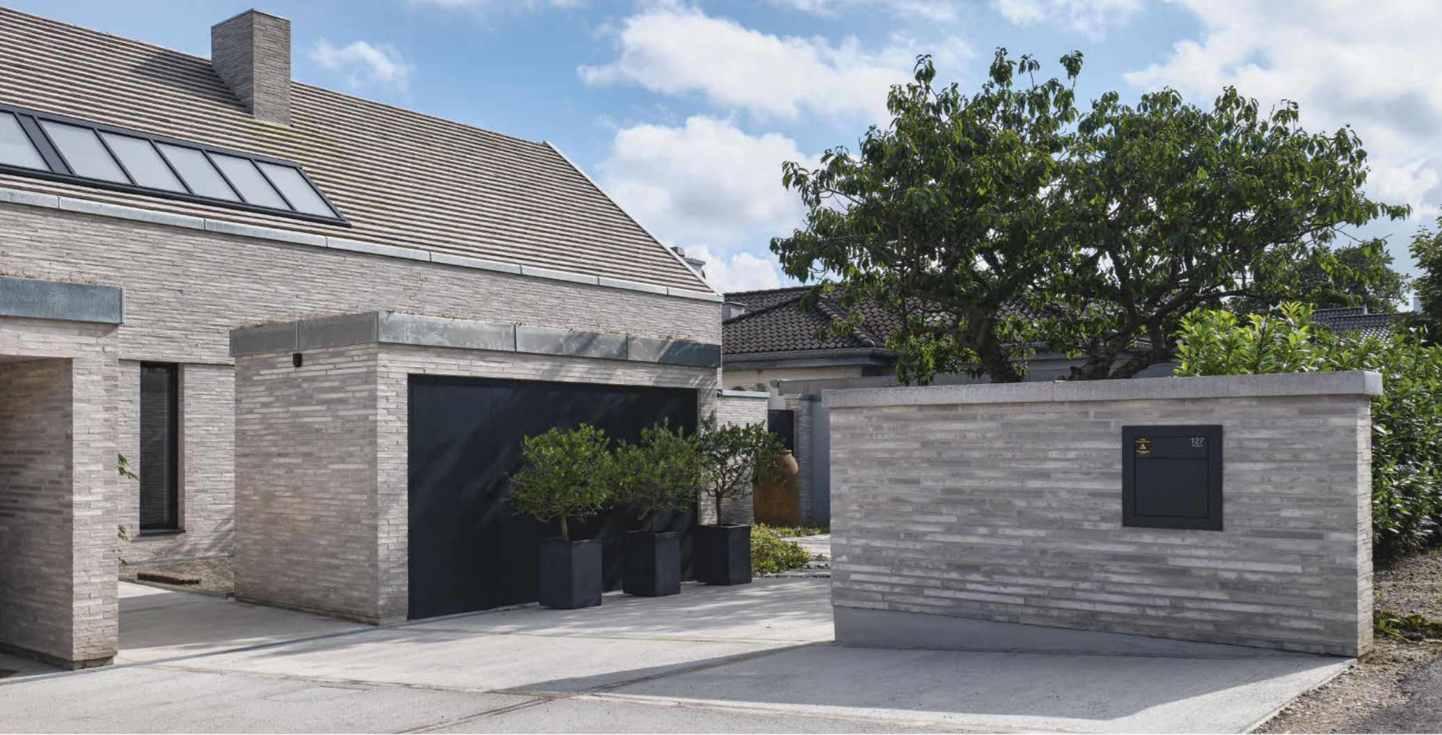
The Kolumba on the façades is also embedded in the grooves in the concrete paving used throughout the arrival area. This detail, and a series of smaller brick structures, help to anchor and root the building.
