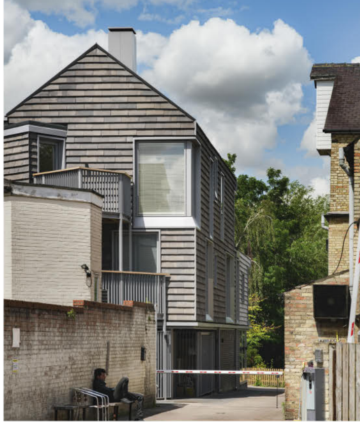
In addition to the aesthetic qualities of the brick, the fact that Cover can be removed and reused almost endlessly played a significant role for the architects and client.
