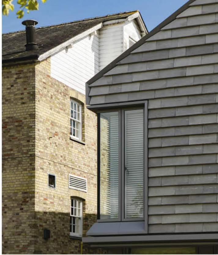
The east wing of Mill House is clad with C54 and C50. Both brick shades are found in the yellow brick façades on the neighbouring Newnham Mill, originally built in 1798, but altered over the years.
