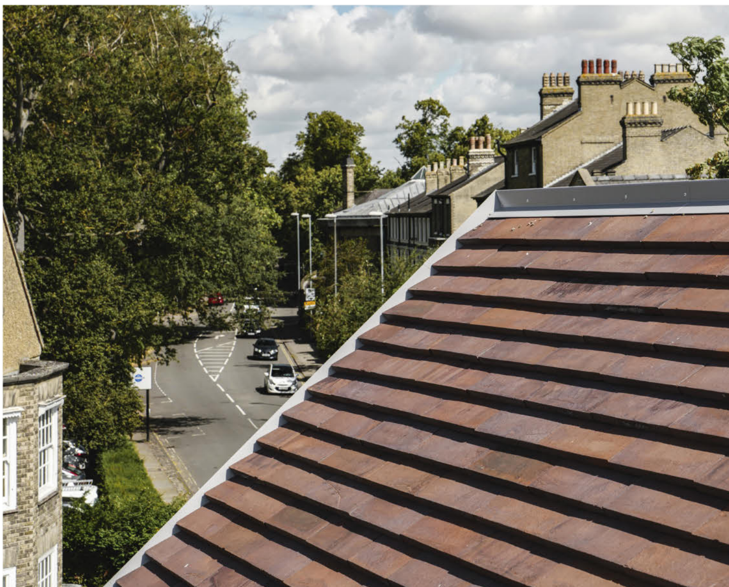
The architects had several options for the corners where the Cover cladding on the roof and on the gable meet the Cover-clad façades. In both cases, MCW Architects chose to run the Cover bricks perpendicular to an aluminium profile. Also the ridge on the roof is finished with aluminium flashing.
