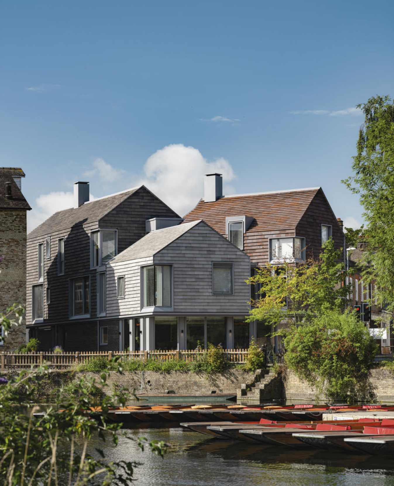
The building consists of a cluster of three smaller volumes. No matter the angle from which they are viewed, they look separate. All three are clad in different versions of Cover, all the colours of which are echoed in the brick façades and tiled roofs of the surrounding buildings.
