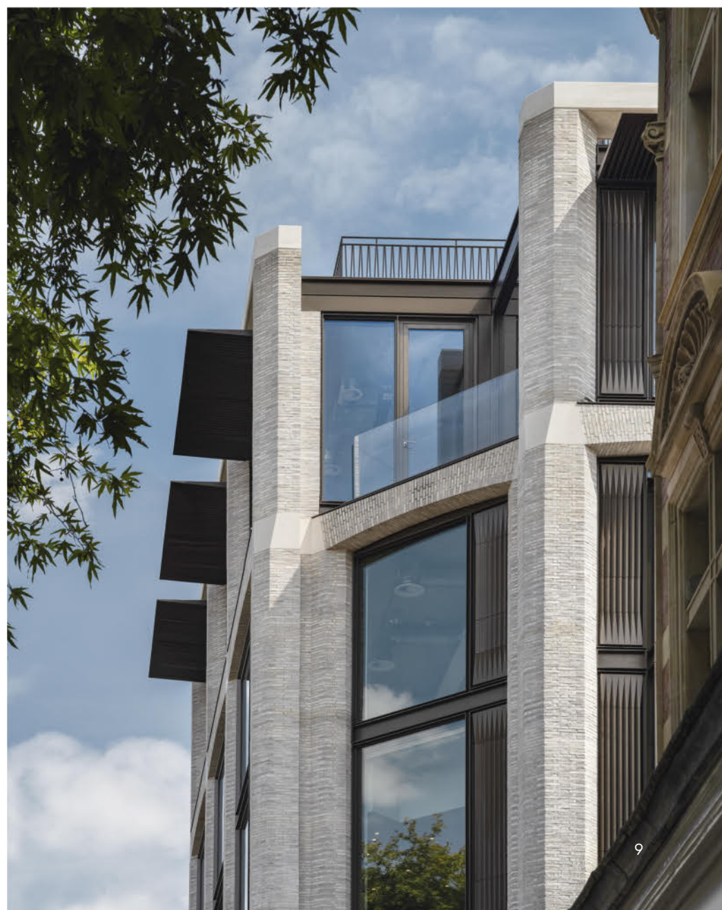
Light-coloured Moleanos stone inserted into the columns marks the different storeys and finishes off the brickwork at the top. Kolumba is laid with a flush joint so that the brickwork follows the façade line of the Moleanos stone.
