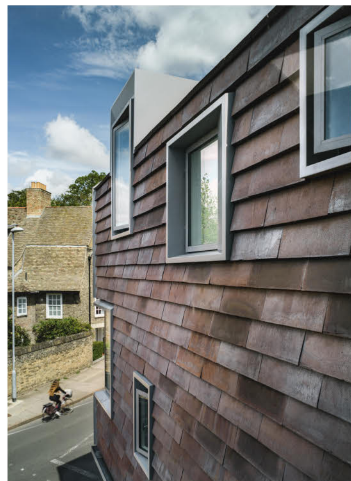
Among other things, the dormers and window surrounds are clad in grey-powder coated aluminium, all custom-made.
