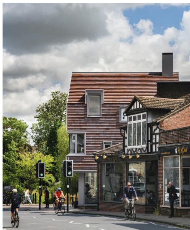
The chimneys are visually important and are used for ventilation.
