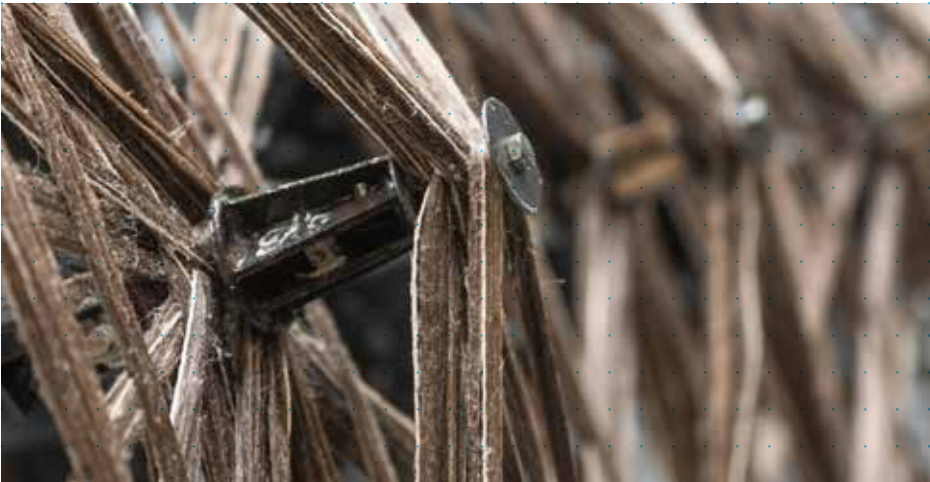
Robotic winding of flax-fibre ceiling
