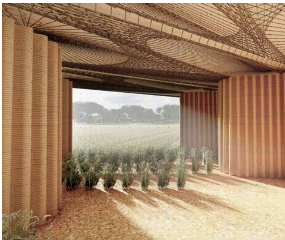
Speculative design for a building combining earth printing with a natural fibre-wound structure (ITKE and IAAC 3DPA)
