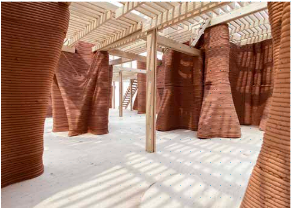
Speculative design for a construction system combining earth with a timber structure (IAAC 3DPA)
