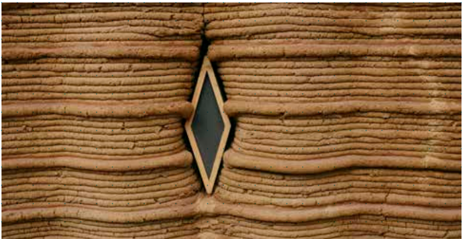
3D-printed earth wall with opening
