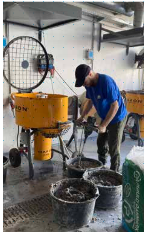
The biopolymer raw material is mixed pre-printing with common construction tools.
