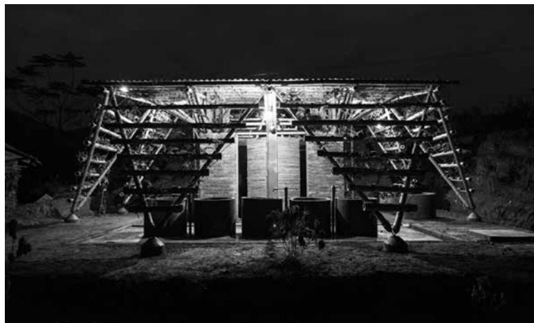
4 Toigetation is featured as a case study contributing to SDG 6. It is a bathroom and washing facility constructed in Son Lap Commune, Bao Lac, Cao Bang Province, Vietnam. The project follows three objectives: quick construction, low cost, and replicability. Designed by H&P Architect led by Dr Nguyen Tri Thanh with the Son Lap Commune and volunteers.
