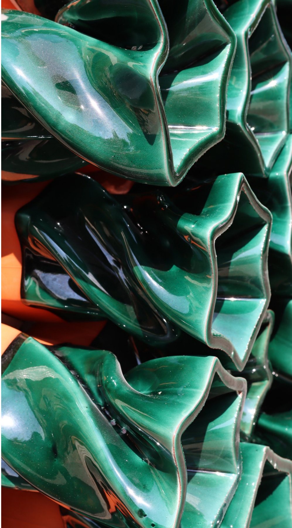
14 Resulting tile assembly as an expressive, color-clay-based building ventilator.
