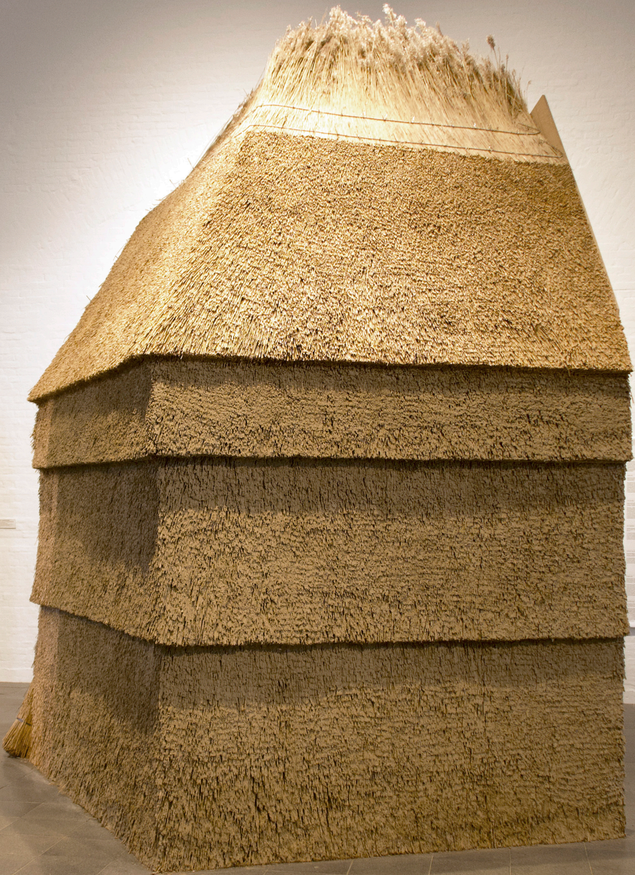
Example of a Materials strategy for an exterior wall construction covered with reed/thatch treated with clay for fire protection. 9
