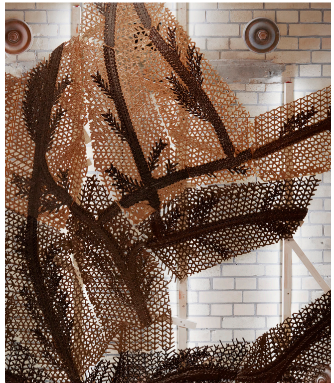
2 Radicant: A 3D-printed biopolymer composite wall paneling system. The panels are composed of interlacing print beads and varying material recipes
