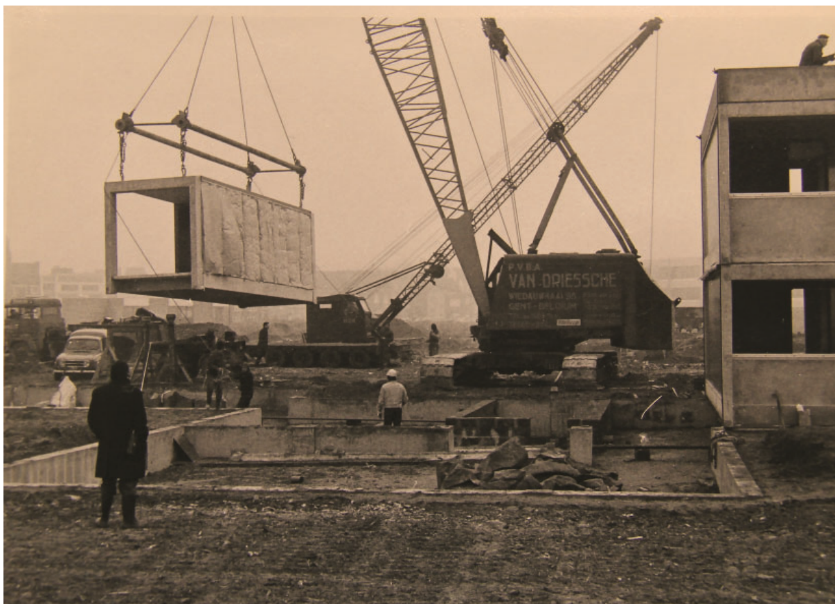
Fig.1, Delivery of the modular units for the construction of the student homes at the VUB campus in Elsene in 1973 – © Archive of the Technical Service 'Infra' of the Vrije Universiteit Brussel.
