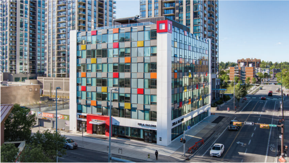
Fig.1, Cube, an office to residential conversion in Calgary, AB - source unknown
