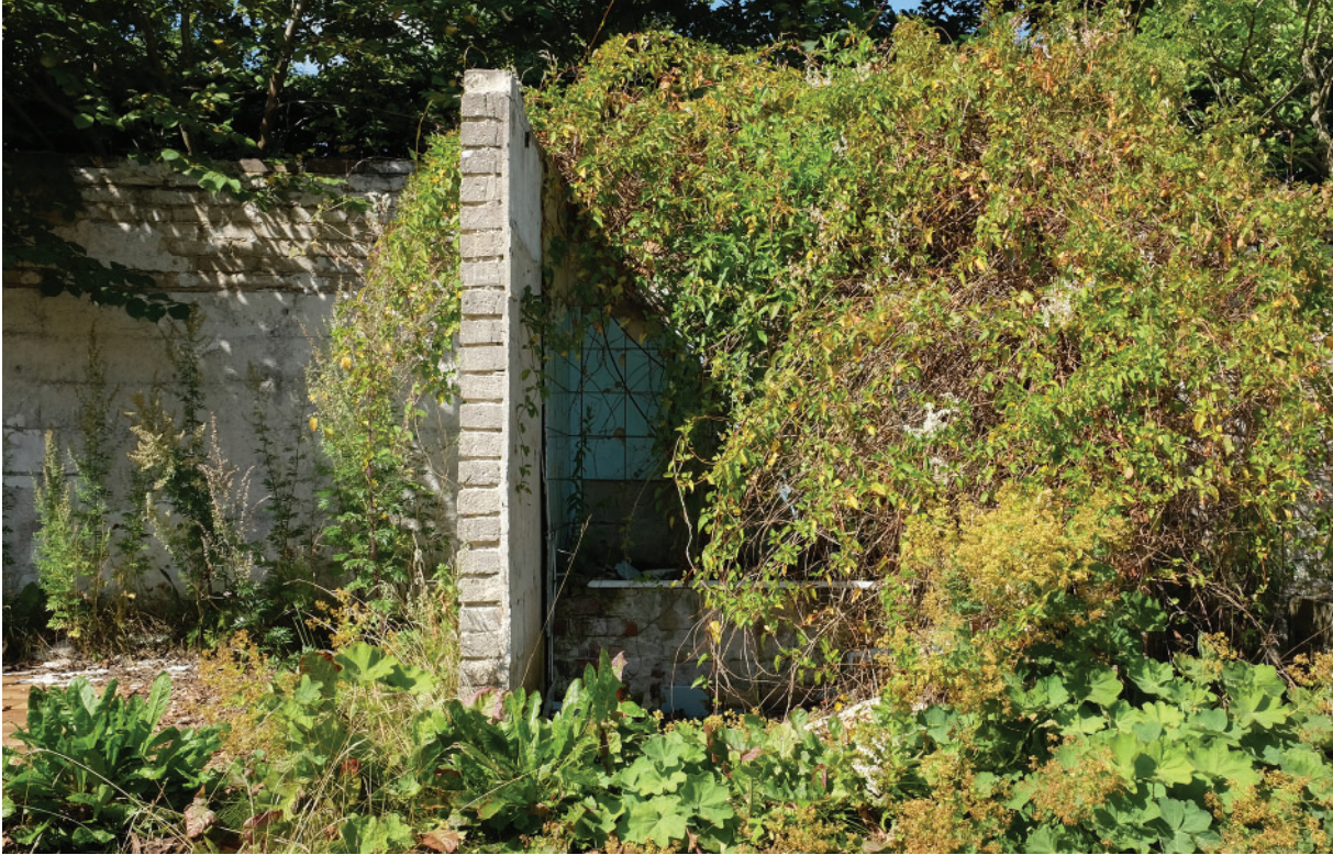
Fig.1, Preservation-prototype eight years after implementation (photograph by author)
