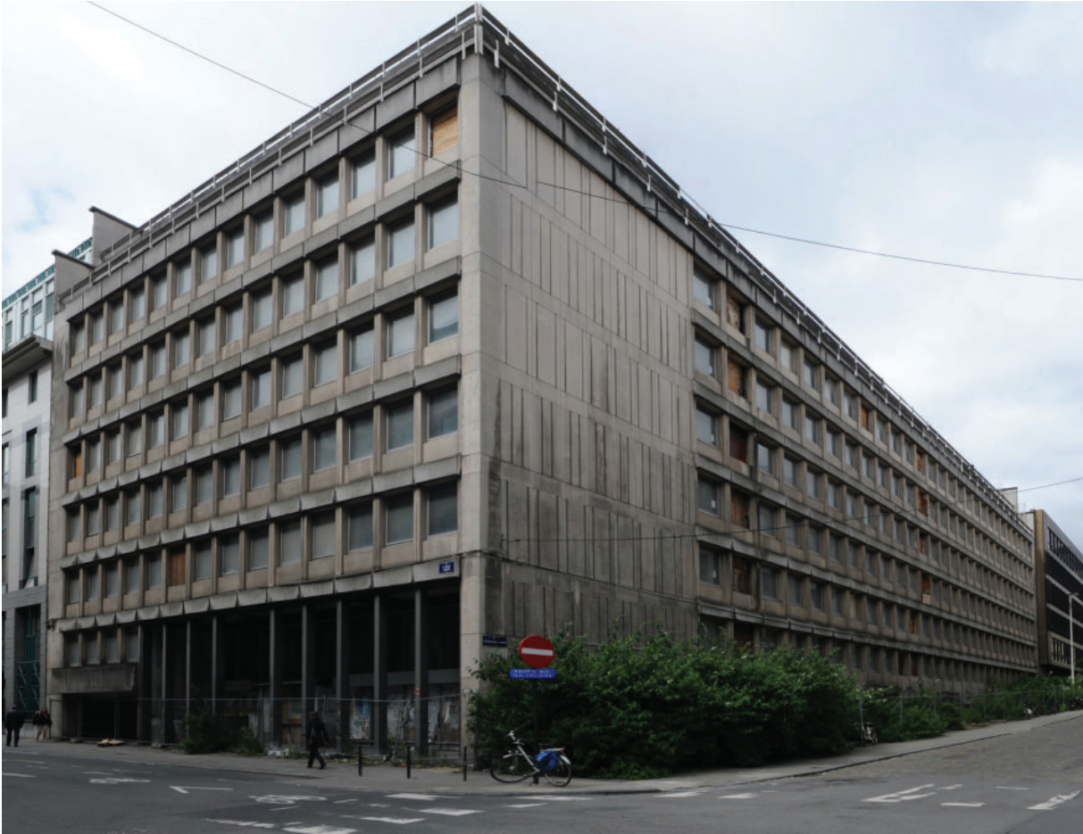
Fig.1, Arlon 104 building – Photograph Philippe Waldner
