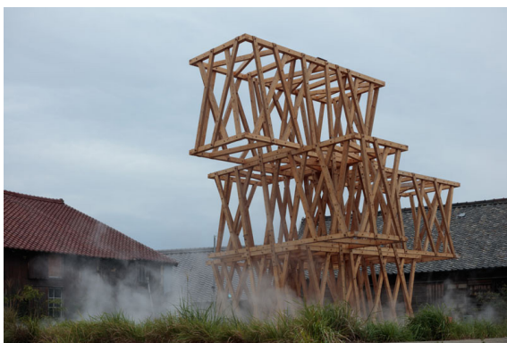
Fig 2.6 Robotically assembled timber-only jointed structure on-site in Japan 2019-22 © Gramazio Kohler Research, ETH Zurich.
