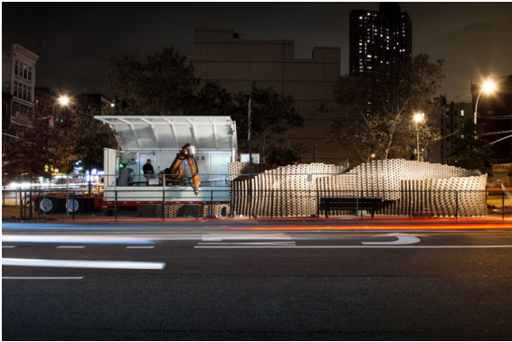
Fig 2.10 The R-O-B setup on-site in New York, USA, 2009 to assemble the Pike Loop project © Gramazio Kohler Research, ETH Zurich.
