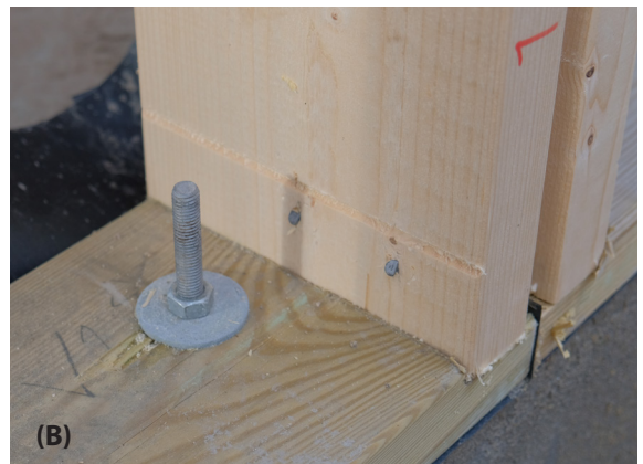
Fig 3.5 Besides the floor separating detail in fig 3.3, the project developed two other details to aid in assembly. A) Details of the notches made for the Olaf Ryes Gade project, which acted as positional information. B) a little groove that was cut for carpenters to rest their nail gun on.
