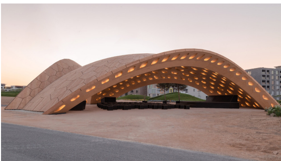
Fig 2.11 The Buga pavilion is a research pavilion made out of LVL cassettes from a near-site robotic process, Bundesgartenschau Heilbronn, Germany, 2019, © ICD/ITKE/IIGS University of Stuttgart.
