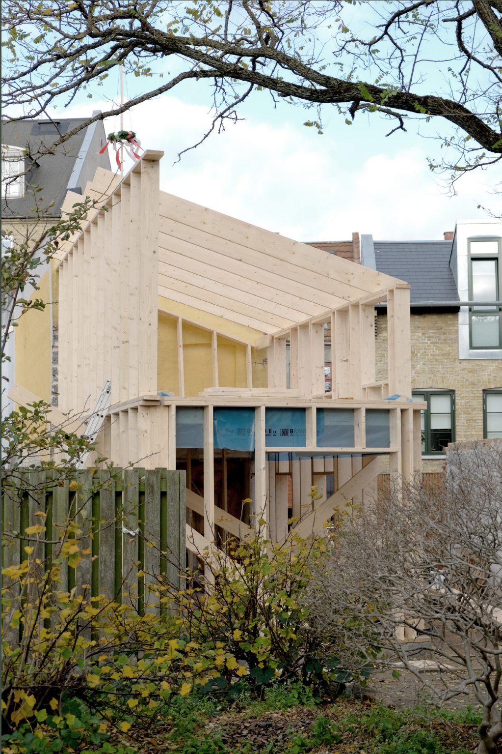
Fig 3.1 The developed construction system on the construction site, 2020, Odense, Denmark.
