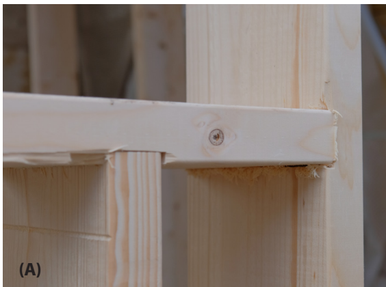
Fig 3.5 Besides the floor separating detail in fig 3.3, the project developed two other details to aid in assembly. A) Details of the notches made for the Olaf Ryes Gade project, which acted as positional information. B) a little groove that was cut for carpenters to rest their nail gun on.
