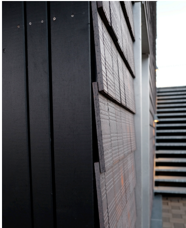
Figure 1. Photo showing the façade detail of the shingles turned inside out. (Photo: Anne Beim)
