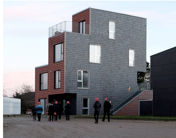
Figure 1. Photo showing the façade detail of the shingles turned inside out. (Photo: Anne Beim)
