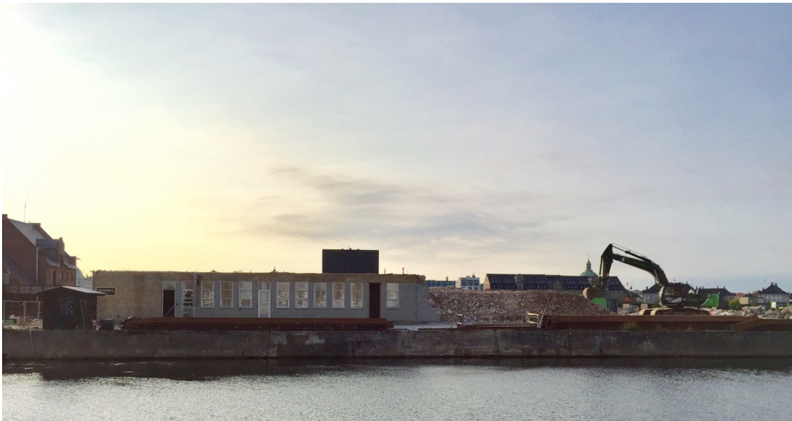
Figure 1. Demolition in process. Photo courtesy: Anne Beim
