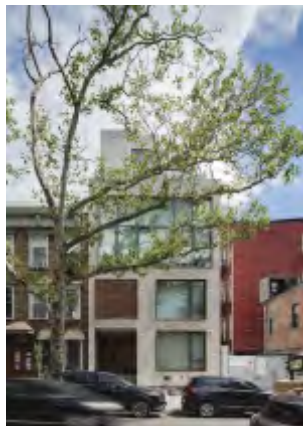
22 113 North 9th Street, Brooklyn Architect: Infocus Completed: 2022 Brick: K91 Photo: Florian Holzherr
