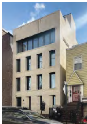
18 84 Meserole Avenue, Brooklyn Architect: Infocus Completed: 2022 Brick: K11 Photo: Michael Sheridan
