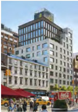
06 345 West 14th Street, Manhattan Architect: DDG Partners Completed: 2017 Brick: K91, D91 FF Photo: Tom Eckerle See Petersen Magazine no. 29
