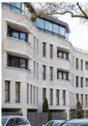
34 280 Marks Avenue, Brooklyn Architect: DXA Studio Completed: 2016 Brick: K11 Photo: Dean Kaufman
