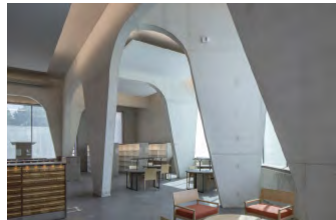
To encourage concentration, the inside of the building offers only limited views of the outside world. Top: The double-height arrival hall. Below: The library reading room. Photos: Paul Kozlowski
