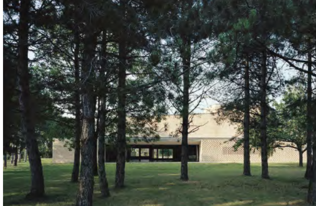
To the south, the cultural centre opens onto a green landscape and a small grove of trees. A covered terrace forms a long niche next to the main hall, acting as a transition between inside and outside. Photo: Audrey Cerdan
