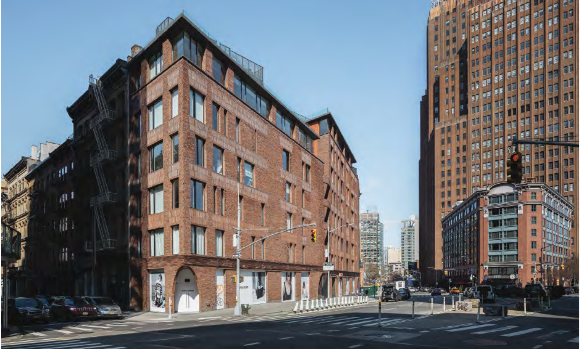
100 Franklin Street in TriBeCa consists of two buildings, one with six storeys and one with eight, separated by a courtyard. Facing 6th Avenue, the two buildings are connected by four brick brackets shaped to follow the curve of the avenue.
