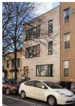
25 264 North 6th Street, Brooklyn Architekt: Infocus Fertiggestellt: 2022 Ziegel: K11 Foto: Michael Sheridan
