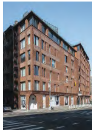
20 100 Franklin Street, Manhattan Architekt: DDG Partners, HTO Architect and Palette Architecture PLLC Completed: 2018 Brick: K4, K33, K43, D33 FF, D43 FF Photo: Dean Kaufman See article on page 5
