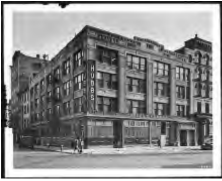
The project included the restoration and remodelling of a 1916 industrial building.
