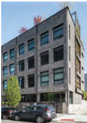
24 59 South 4th Street, Brooklyn Architect: Arcus Design Group Completed: 2015 Brick: D54 FF Photo: Dean Kaufman See article on page 10
