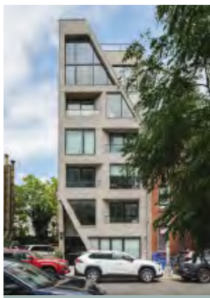
16 141 Green Street, Brooklyn Architect: INOA Architecture Completed: 2018 Brick: K91 Photo: Florian Holzherr
