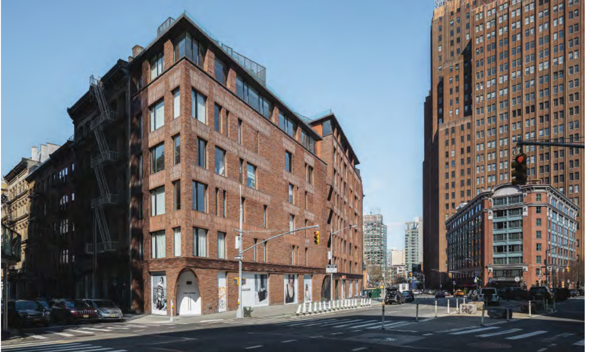
100 Franklin Street in TriBeCa consists of two buildings, one with six storeys and one with eight, separated by a courtyard. Facing 6th Avenue, the two buildings are connected by four brick brackets shaped to follow the curve of the avenue.
