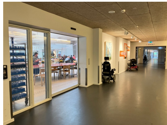
Figure 6.1-30 Vandhalla: transparent partition between the corridor and the canteen
