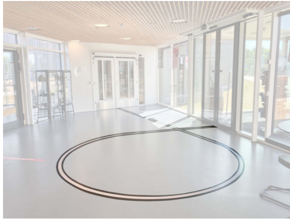
Figure 6.2-9 Musholm: white paving line at the entrance
