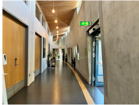
Figure 6.1-17 Musholm: wood guiding line on the floor
