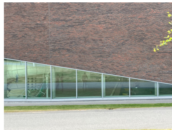
Figure 6.1-56 Vandhalla: transparent partition between the exterior and the swimming pools
