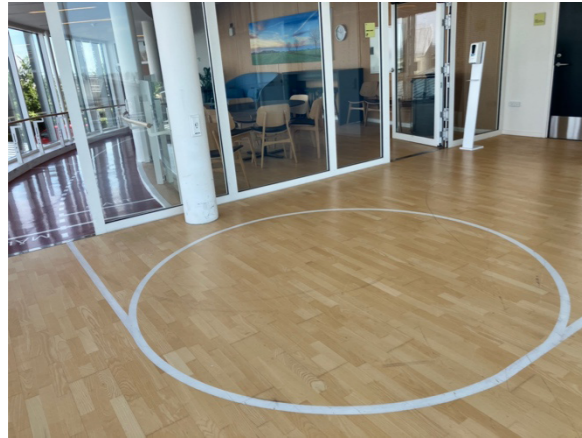
Figure 6.1-16 Musholm: white guiding line on the floor at the upper level
