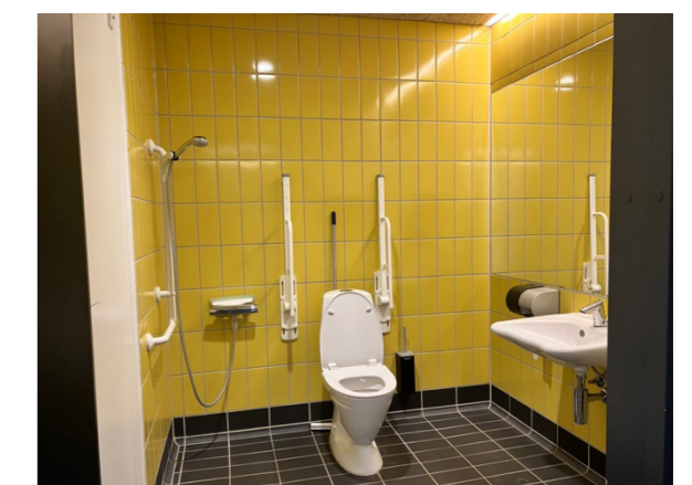
Figure 6.1-10 Vandhalla: coloured tiles in contrast with the accessories and sanitary facilities
