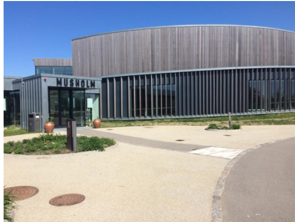
Figure 6.1-3 Musholm: contrasting colours and tactile surfaces of the external paving
