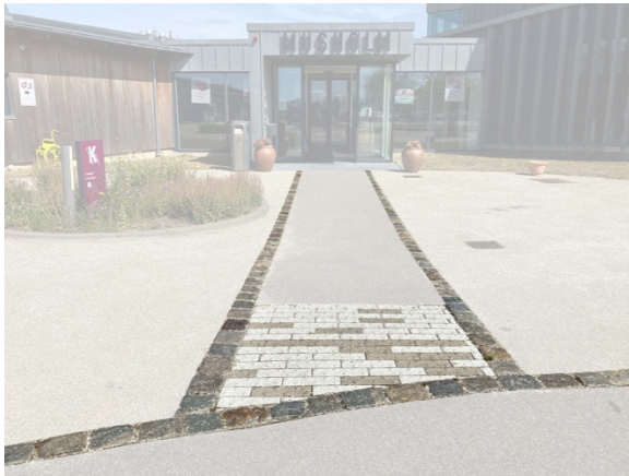
Figure 6.2-4 Musholm: tactile surfaces of the external paving
