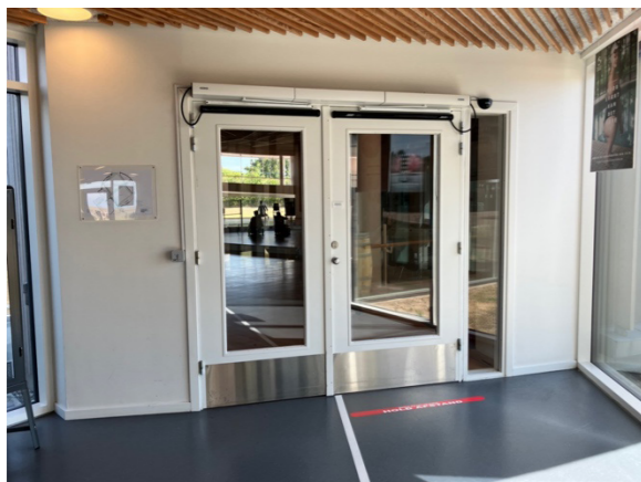
Figure 6.1-32 Musholm: transparent partition between the en- trance and the multi-purpose hall
