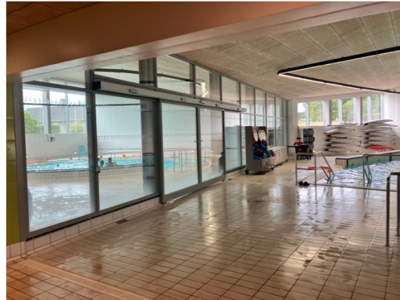
Figure 6.1-28 Vandhalla: transparent partition between the two swim- ming pools
