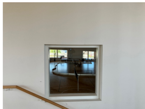
Figure 6.1-33 Musholm: transparent partition between the ramp and the mul- ti-purpose hall
