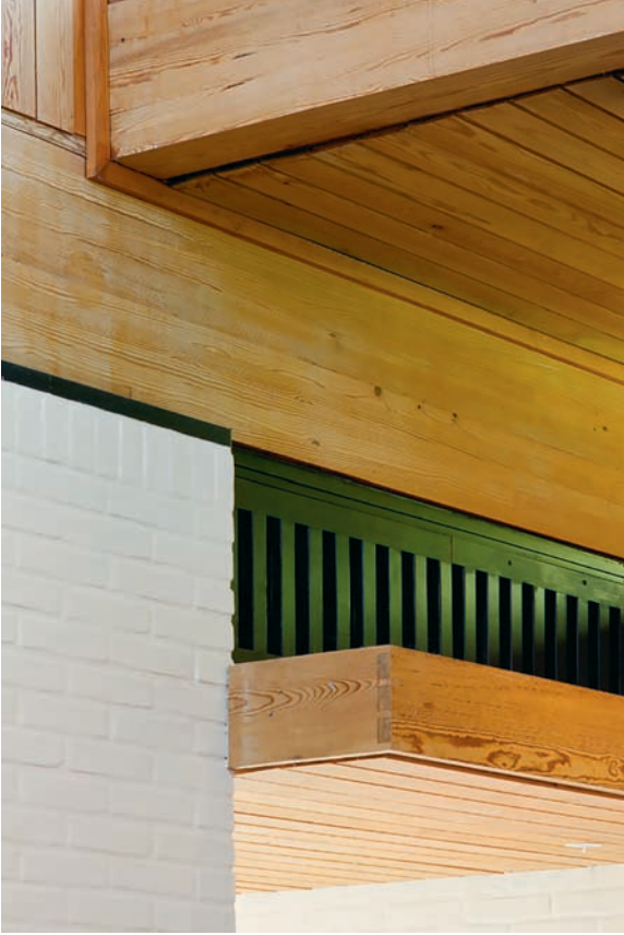
2.59 Intersection of elements at entrance to first Lantern Gallery. The ceiling in Tree Passage extends into the gallery, to reinforce the sensation of continuous space.
