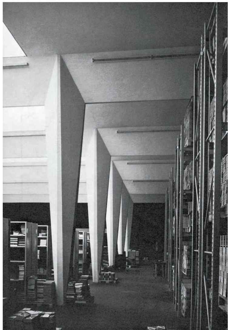
3.42 Gyldendal warehouse, packing hall with faceted concrete structure and skylights.
