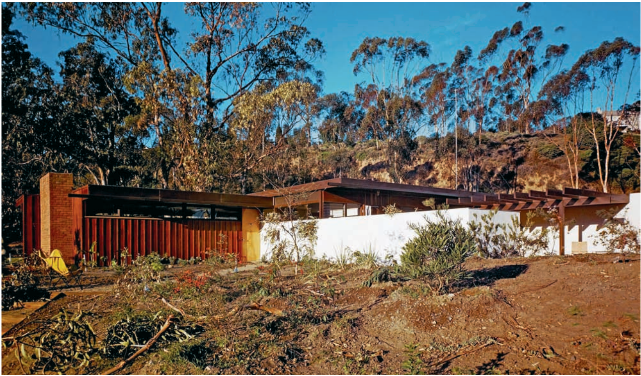
1.44 CSH #20. Exterior view towards entrance and white walls enclosing work patio with carport.
