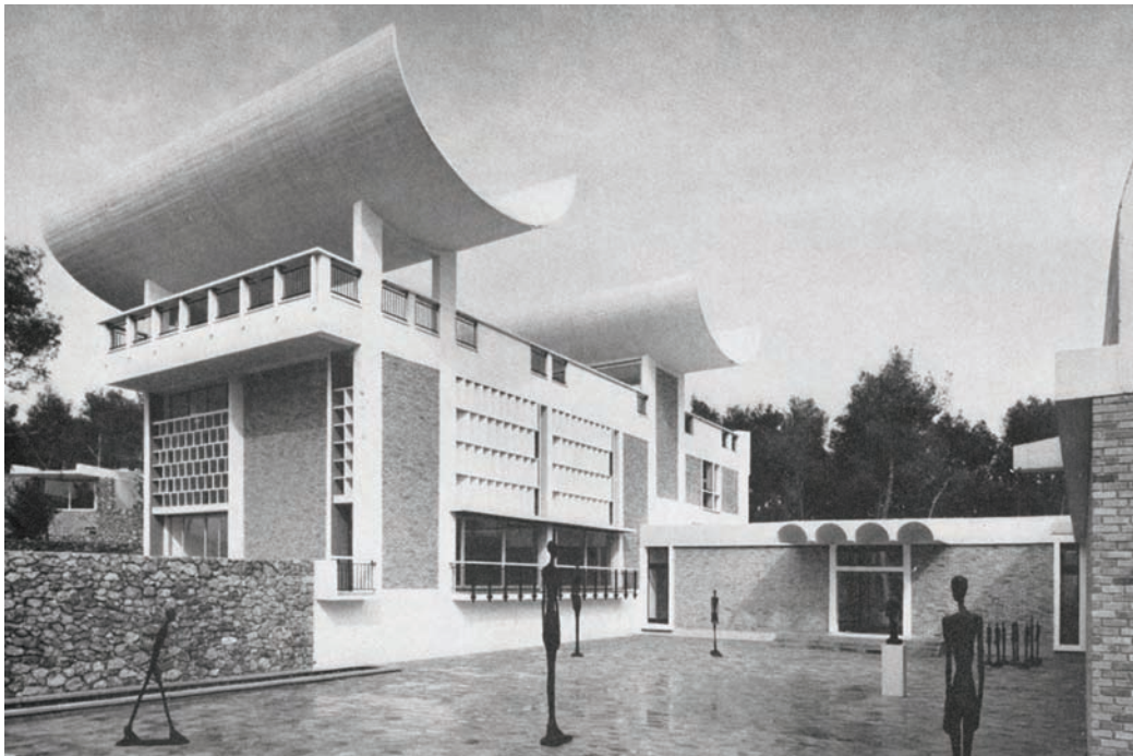
3.84 View of the Town Hall from La Cour Giacometti , with entry structure in background and a corner of the Cloister.
