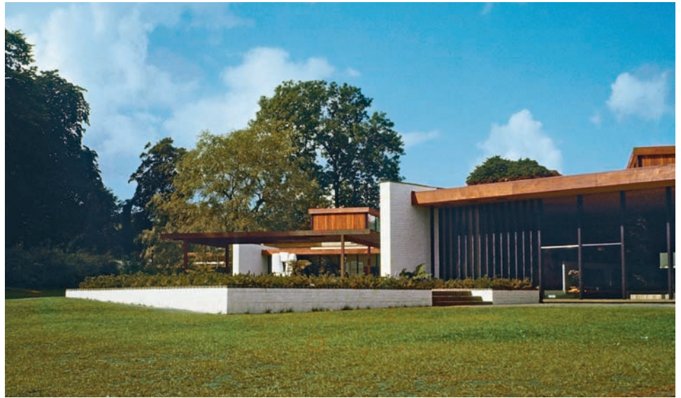
2.46 Terrace in front of library, with pergola and lantern galleries beyond.
