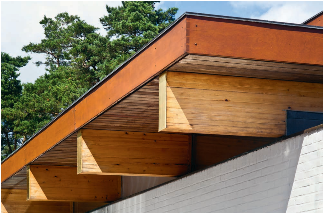
2.61 Detail of roof structure at lantern galleries, with gold-leaf covering plates and dovetail joint on fascia.
