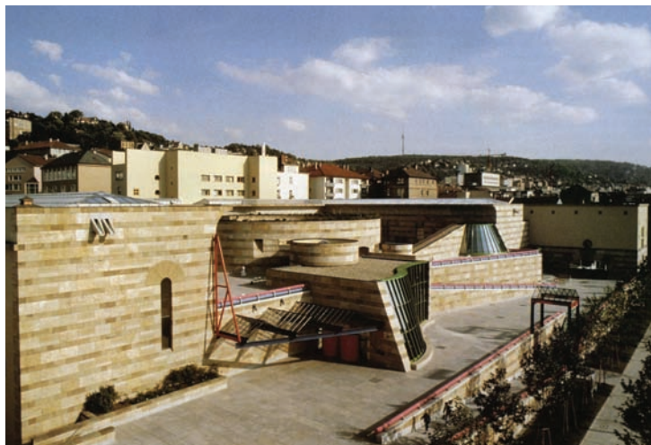
4.95 Neue Staatsgalerie. View of terrace along Konrad-Adenauer-Strasse and main entrance.
