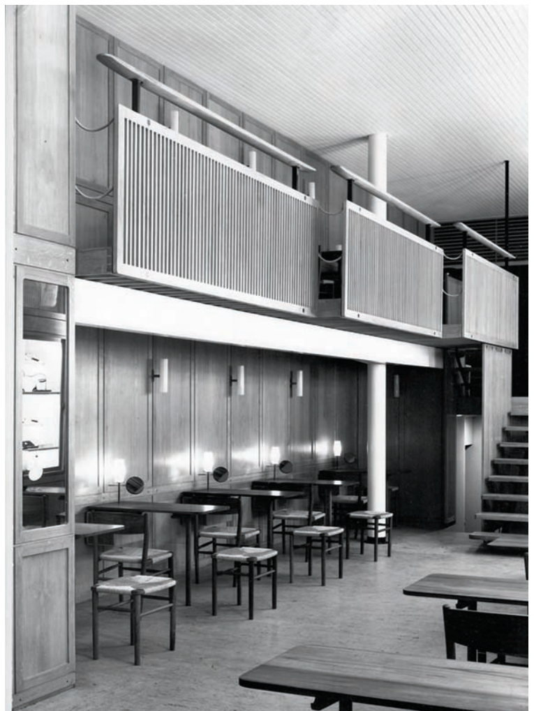
1.57 F. A. Thiele shop. View towards stair and balcony.
