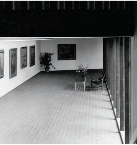
2.27 Entrance to the Tree Passage from north end of the villa.
