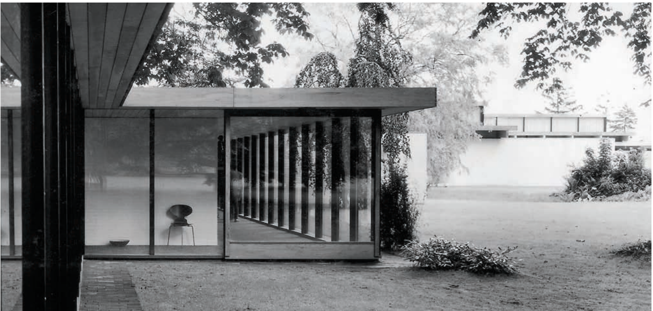
2.29 Third segment of the Tree Passage, seen from the park, with the lantern galleries in the background.
