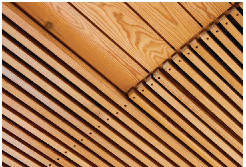
2.51 Detail of acoustic ceiling in the library.
