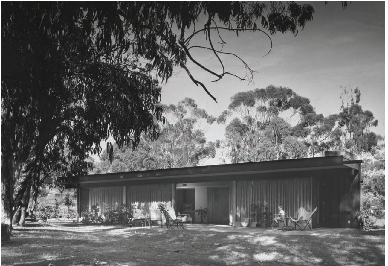
1.47 CHS #20. View from southwest.
