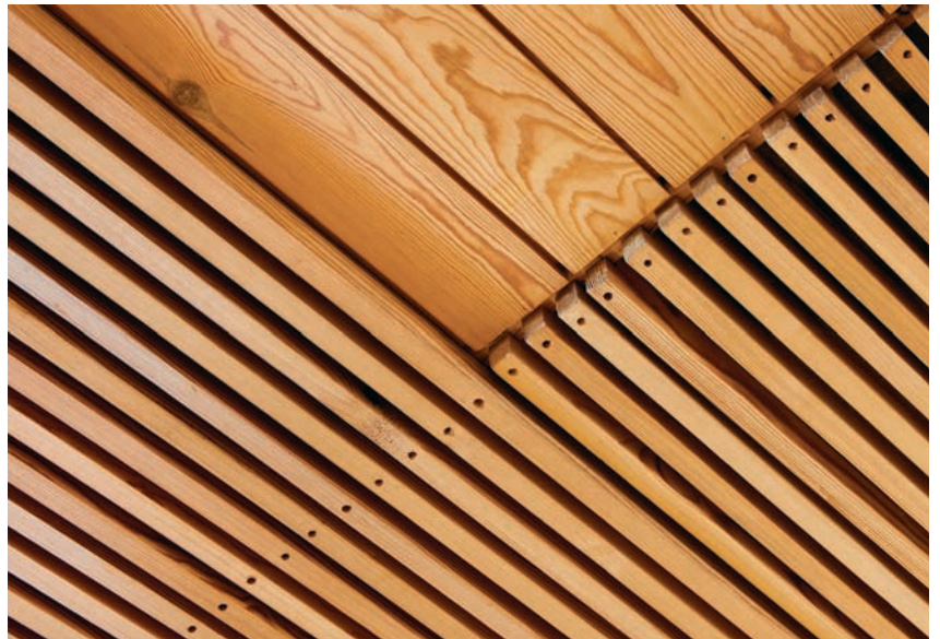
2.51 Detail of acoustic ceiling in the library.
