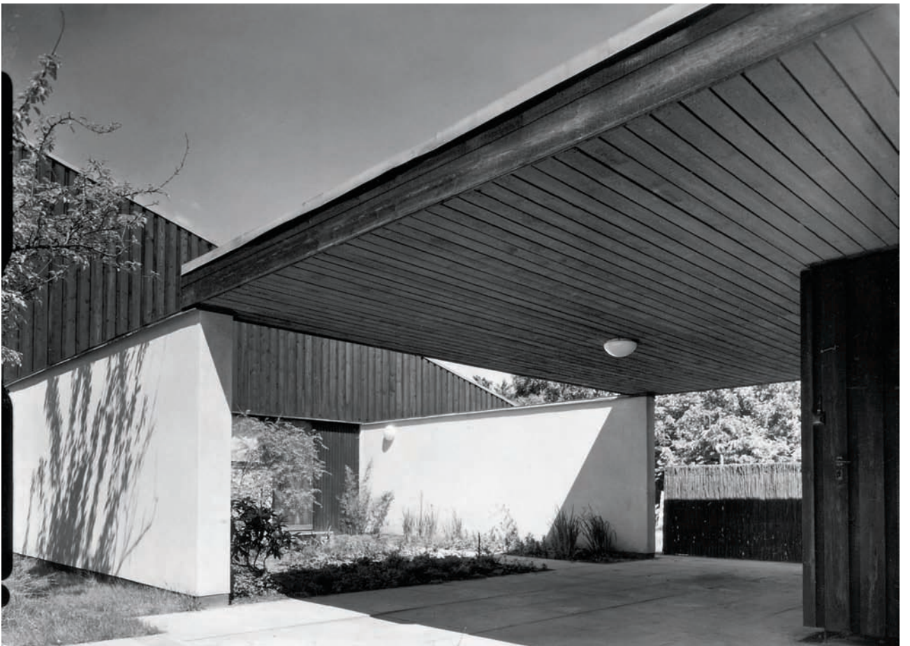
1.51 Bo House. Carport with flower garden and main entrance (left) and passage to children's terrace (right).
