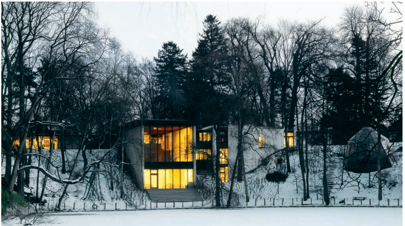
5.36 Children's House. View across the lake with 58-Building in beyond and "Glass House" at right, 1994.
