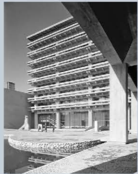
1958 Kagawa Prefectural Office Tange
