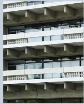
1958 Kagawa Prefectural Office Tange
