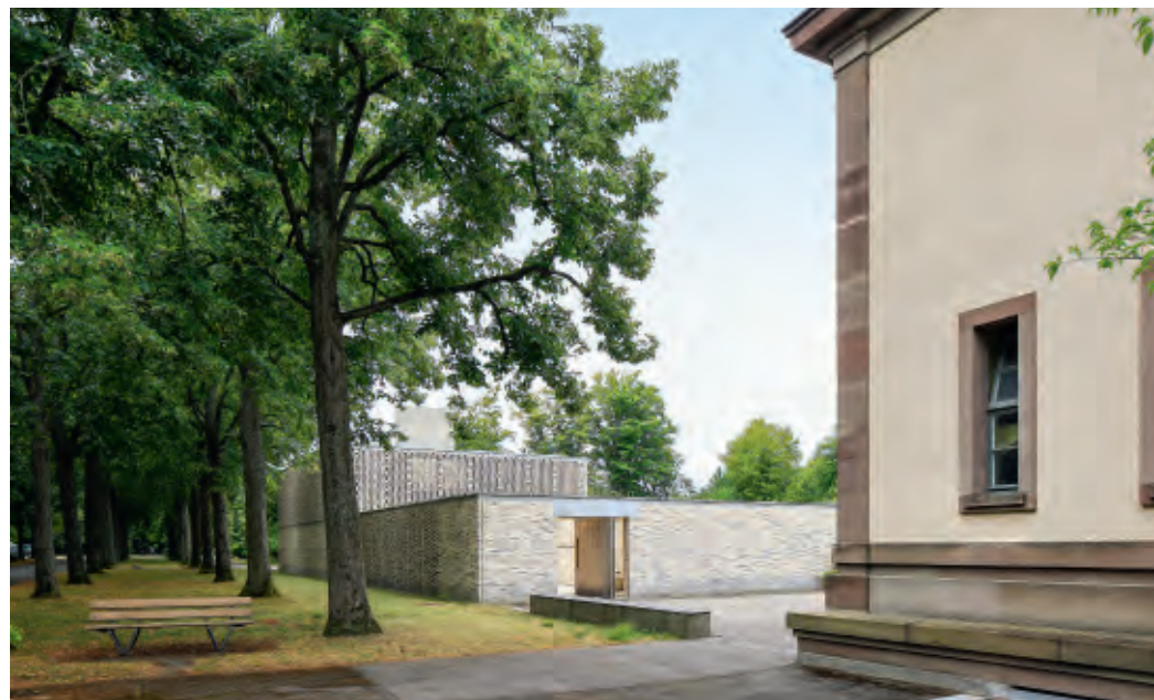
The light, yellowish D71 was chosen because it matches the beige plaster on the older chapel, grey D91 because it fits in with the colour of the decorative sandstone elements.
