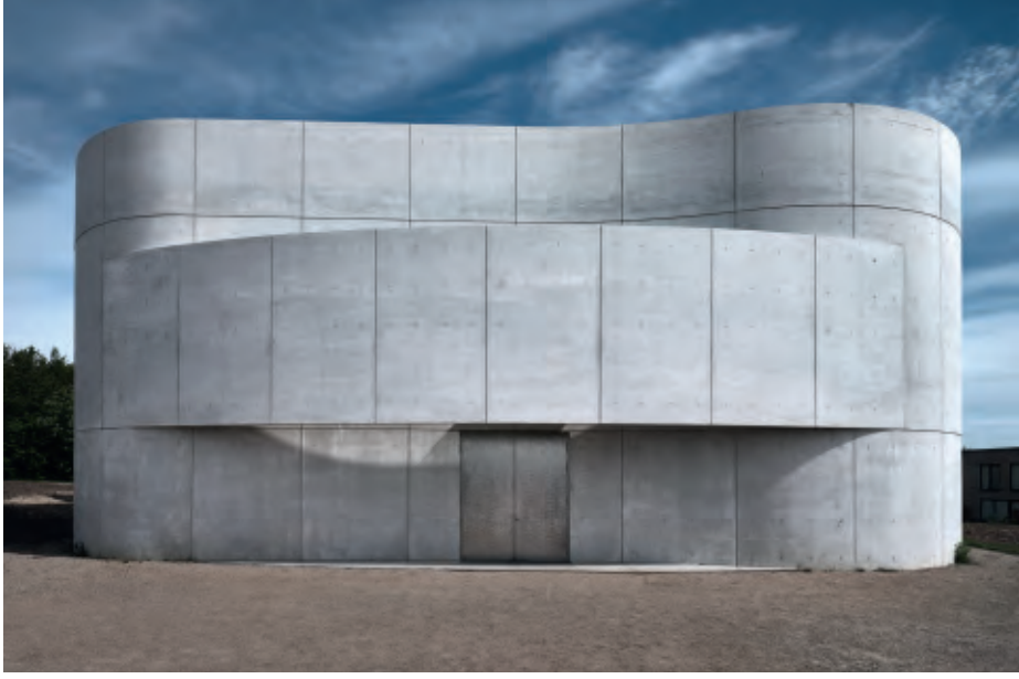
To achieve the organic curves of the church, the contractor produced over 200 moulds to cast the nine concrete sections in situ
