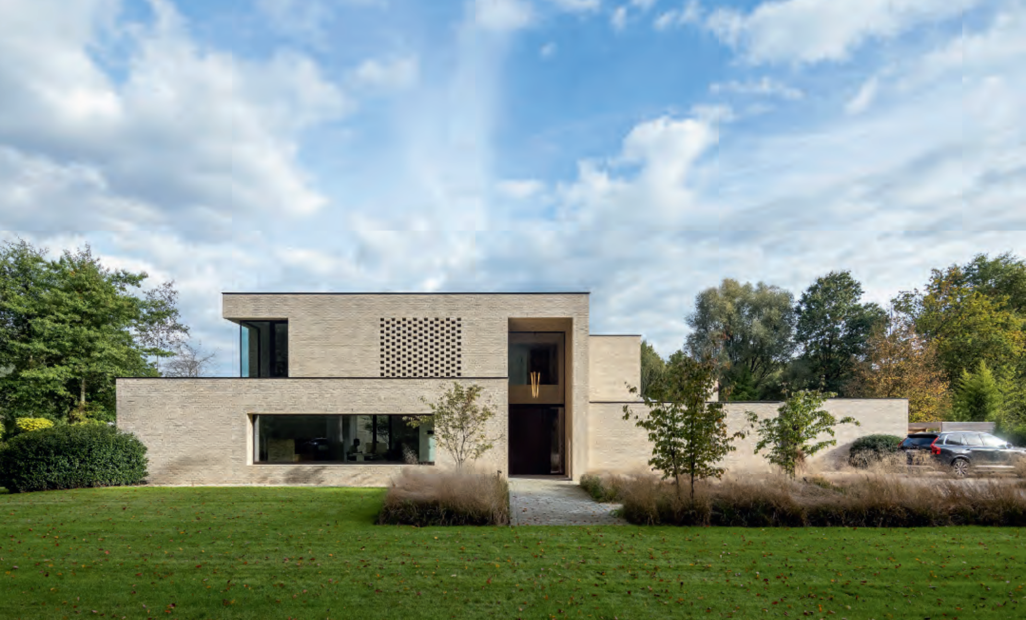
The house near Antwerp consists of interconnected, rectangular volumes offset from each other, both horizontally and vertically. Slightly offset brick pillars, bands and niches add to the variation and spatial depth.
