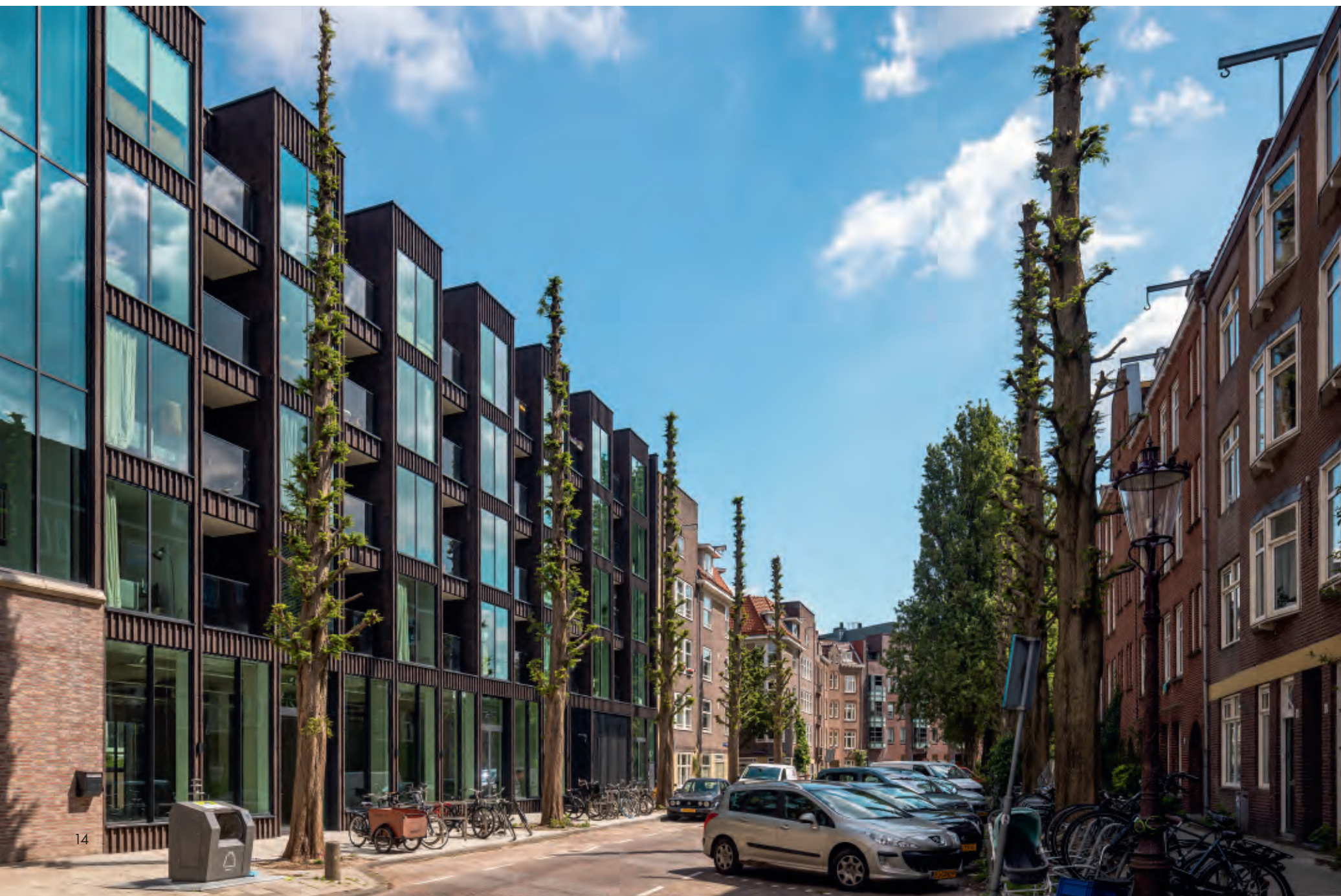
Facing Karel du Jardinstraat, the well-proportioned façade has seven rows of bay windows that run from the first floor upwards, before culminating in a flat roof. Between these rows, balconies have been built into each of the flats.
