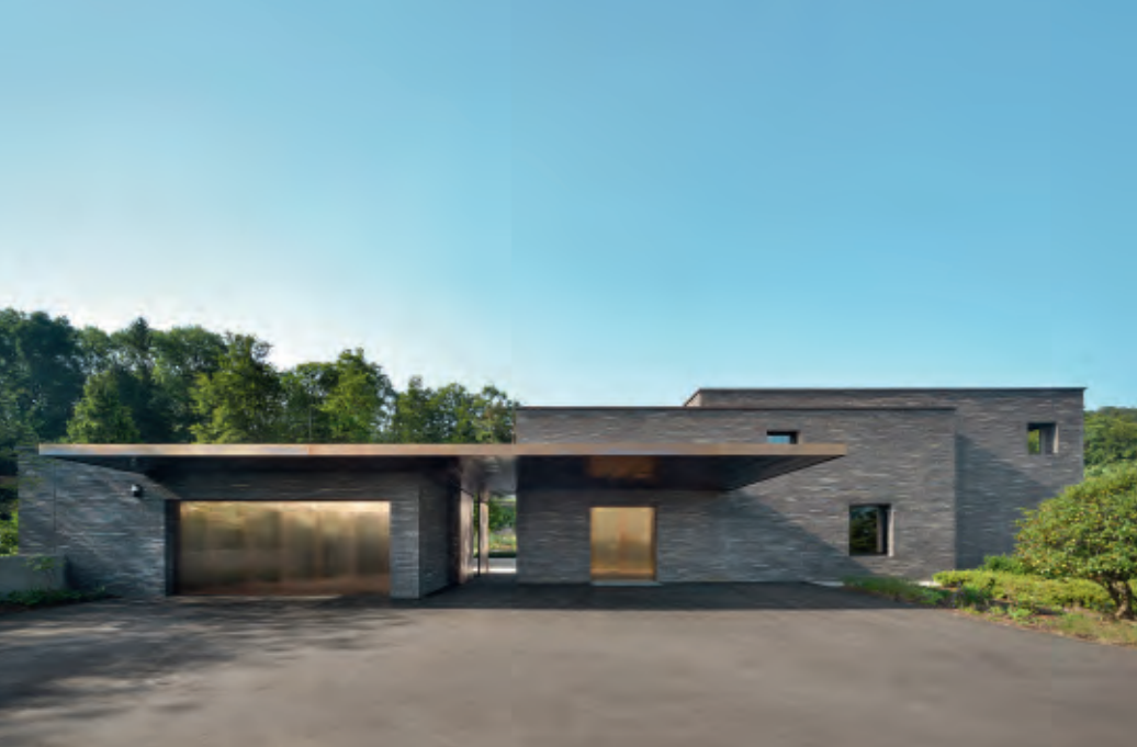
Access to the building and garage is under a large canopy which is clad in copper, as are the door and gate. The layout makes it possible to see the garden from the arrival side.
