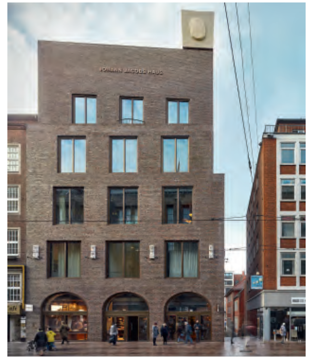
The windows in the building are gathered around the middle. The overall appearance is a subtle reference to Bremen’s historical stepped gables.
