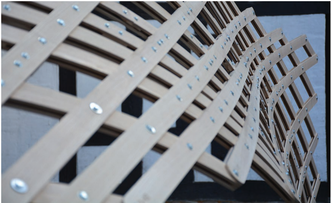
Figure 2.5.21 - Aarhus Geodesic Gridshell, designed and built by 2nd-year bachelor students in June, 2018, under the tutelage of the present author.
