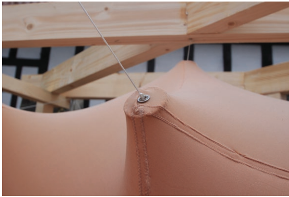
Figure 2.2.23 - Detail of fabric connection
