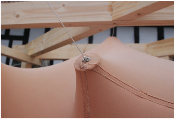
Figure 2.2.23 - Detail of fabric connection
