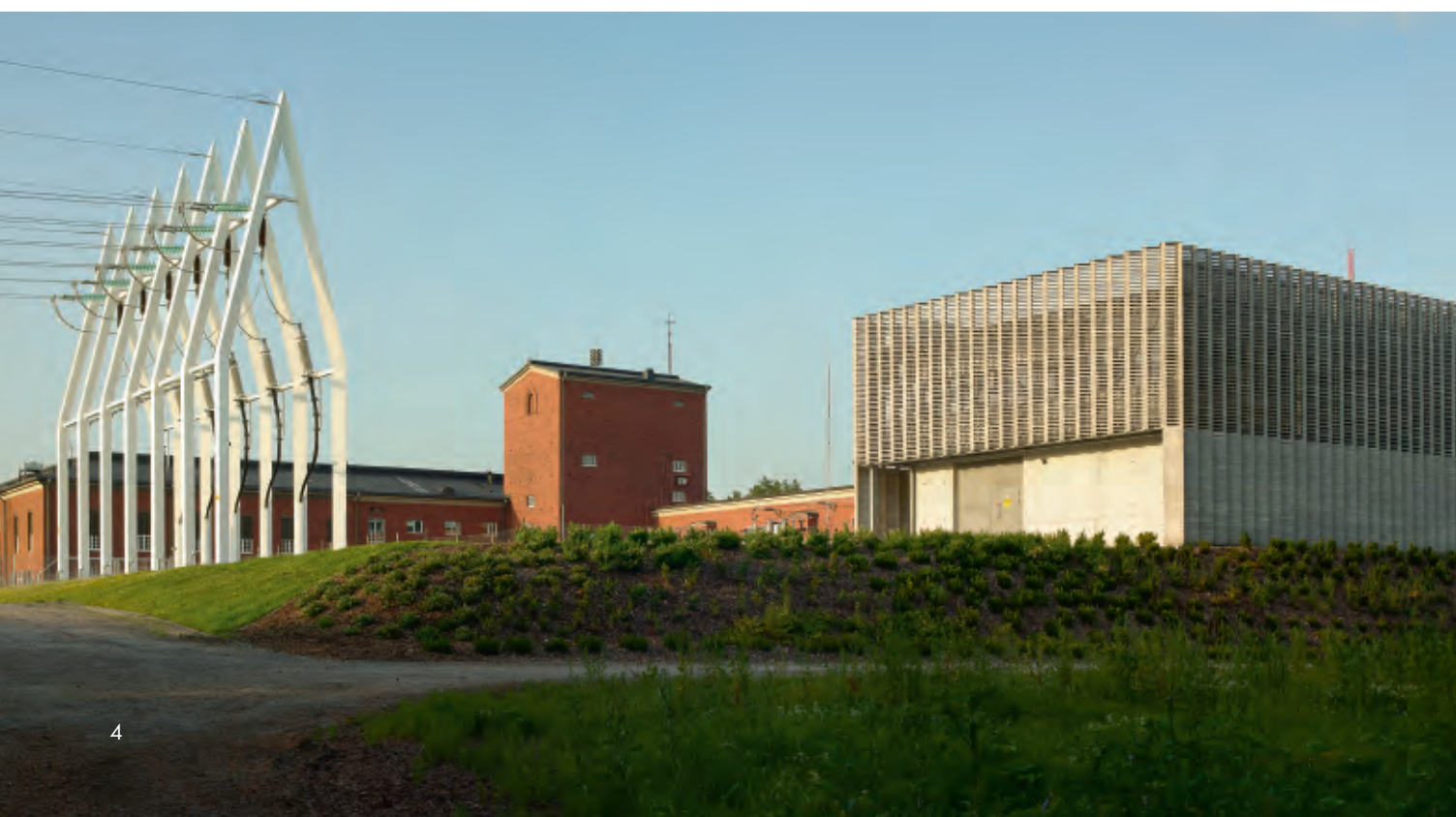
In terms of both scale and location, Imatra Transformer Station has been adapted to fit in with the power plant’s existing buildings. Like the older buildings, it is built in brick, but the architects chose light-coloured stone to match the white-painted steel of the power line structures. Photo: Max Plunger
