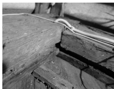
Figure 9: Construction detail at north-western gable. Here, the rafter is made from pinewood and provided with a groove originally intended for the attachment of gable boards. The pinewood rafter is typical to roof constructions and in contrast to the other rafters, presumably made from poplar. Photo, Thomas Kampmann, 2019.
