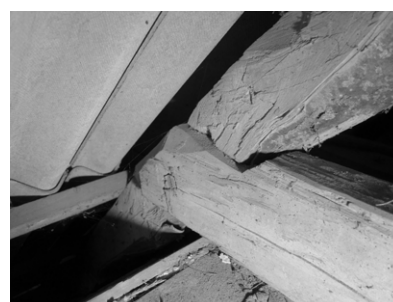
Figure 11: Joint between rafter and collar beams. The rafter and the collar beams are made from the same type of wood. Photo, Thomas Kampmann, 2019. Opposite page top, figure 6: Elevation SW Opposite page middle, figure 7: Section BB Opposite page bottom, figure 8: Plan, ground floor
