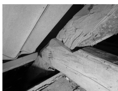
Figure 11: Joint between rafter and collar beams. The rafter and the collar beams are made from the same type of wood.
