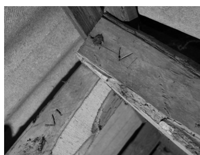
Figure 10: The top joint of rafters in the roof construction in the apprentice house. The timber mark, here on rafter no. VI, indicates a seven-bay house of two gable in pinewood rafters and 6 numbered rafters in between in poplar. Photo, Thomas Kampmann, 2019.
