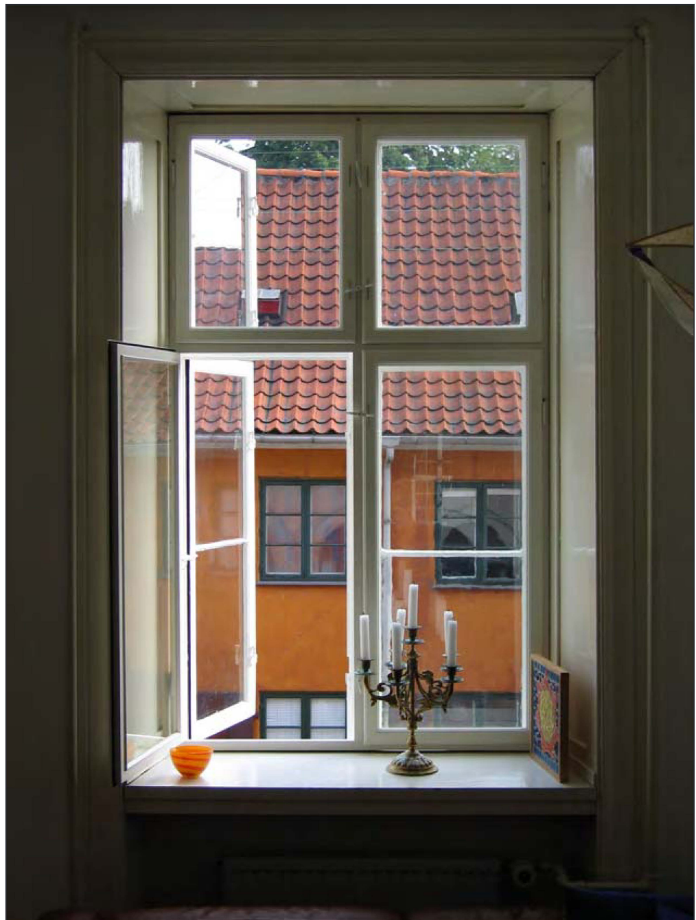
Figure 2. Typical Danish window with secondary glazing. Source: Thomas Kampmann.
