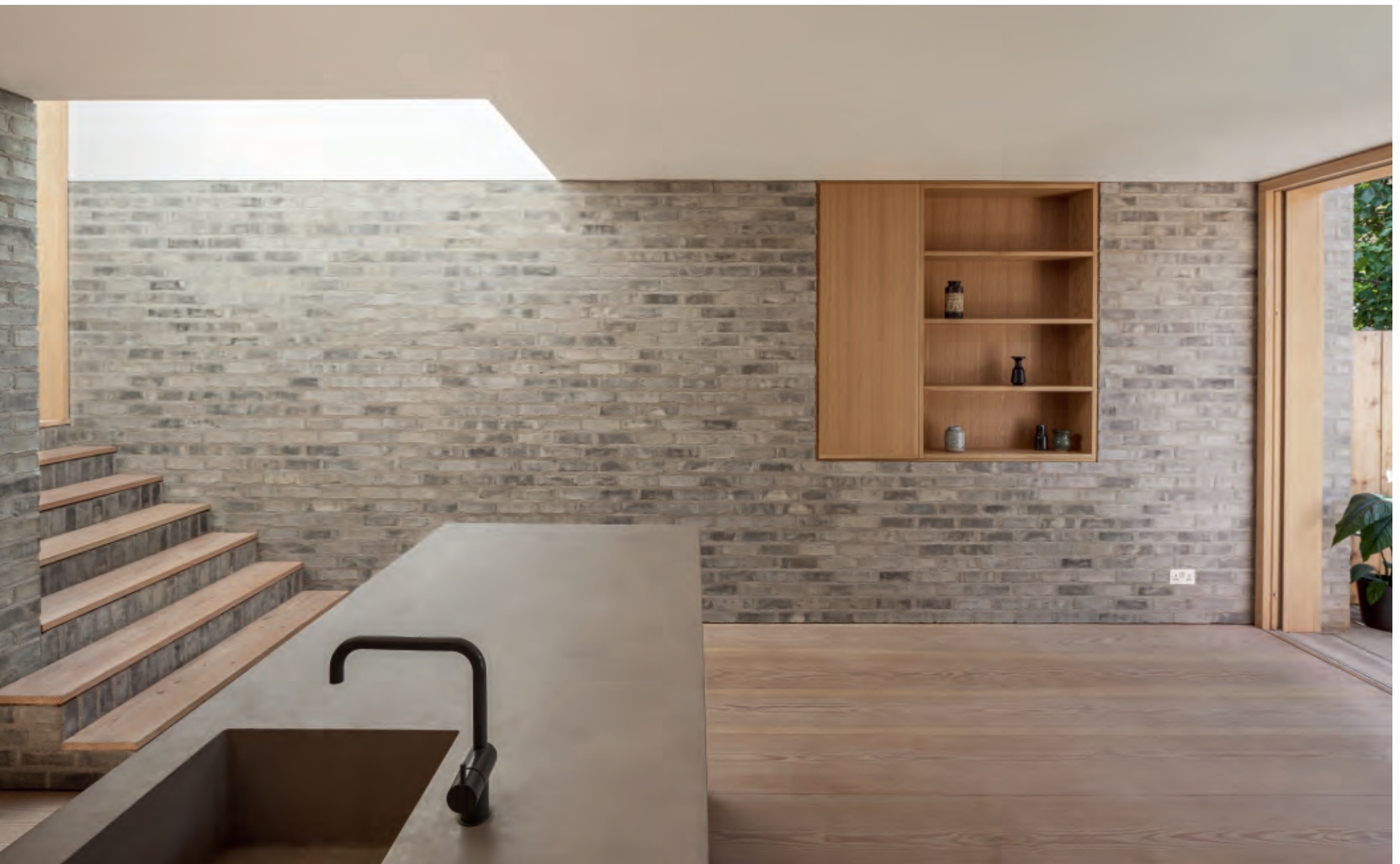
The choice of harmonious materials and colours continues indoors. The floors are clad in lye-treated Douglas fir planks. The shelves and doors are in oiled oak and the kitchen table is made of microcement.
