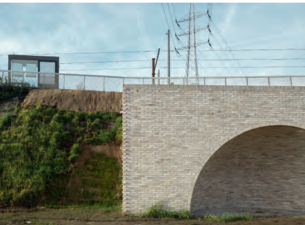
The double-curved brick vaults of the Tjalkstraat substation required consummate skill.
