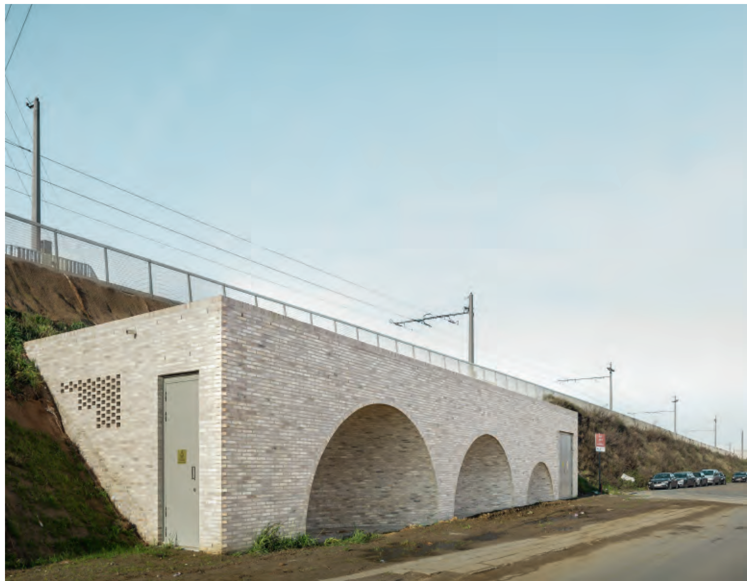
Tjalkstraat substation, with its three double-curved vaults of various sizes, cuts into the embankment on which the trams run.
