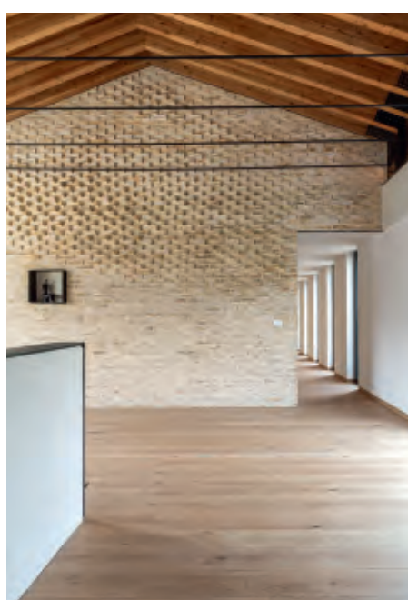
On the end wall of the double-height living space, the bricks are slightly offset from each other, forming an abstract, undulating relief.
