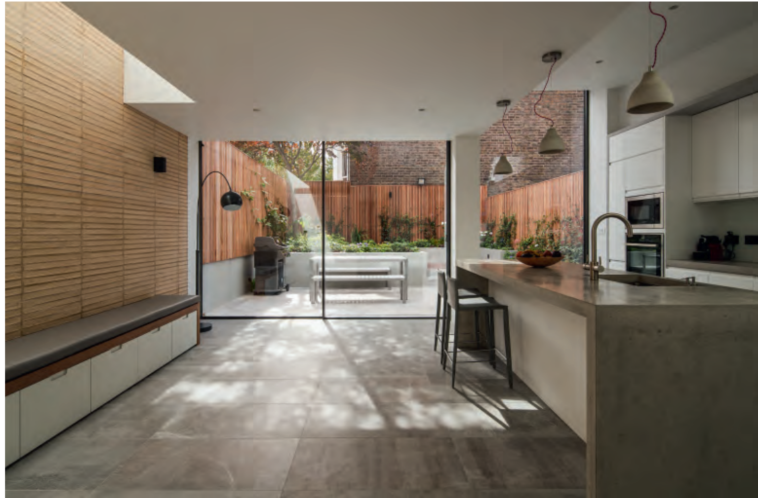
The large wall in handmade, light-coloured Kolumba creates a beautiful contrast to the room's other smooth, cool surfaces, such as the polished stone floor and the kitchen table in polished concrete.
