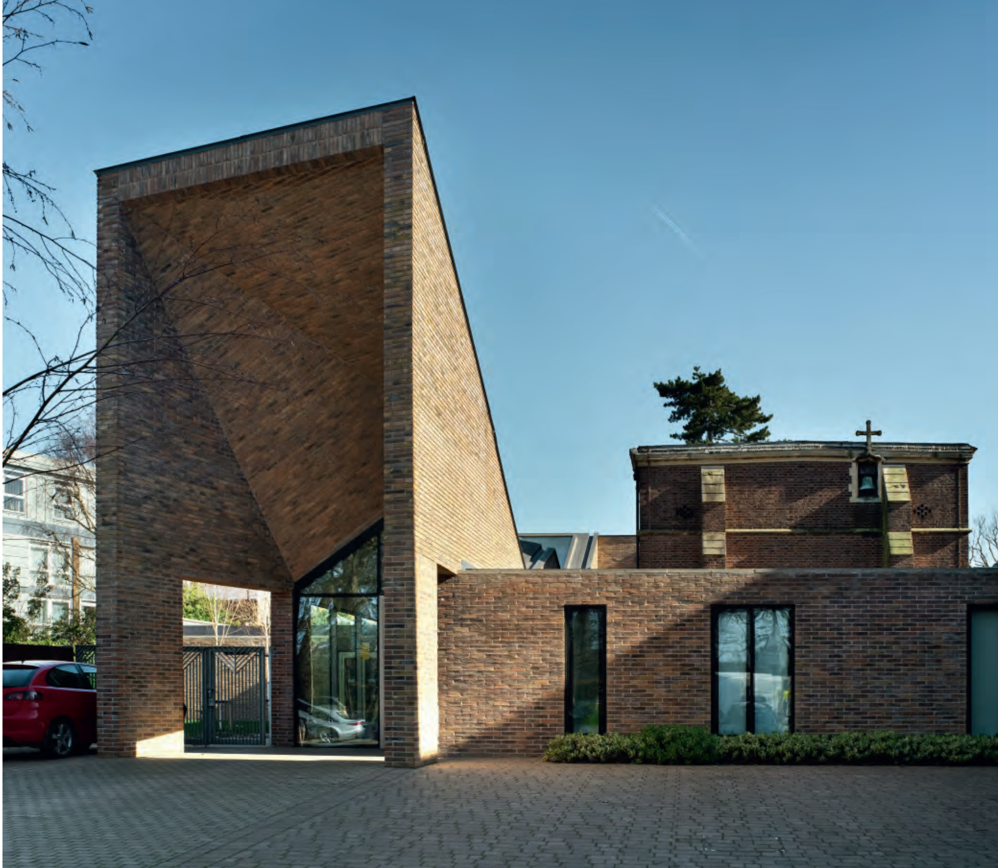
The main entrance consists of an impressive portal formed by the sharp angles in the pleated landscape of the roof surface.
