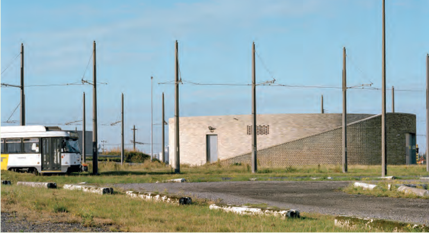
The Straatsburgbrug substation radiates quiet self-assurance amid somewhat less than homogenous surroundings.
