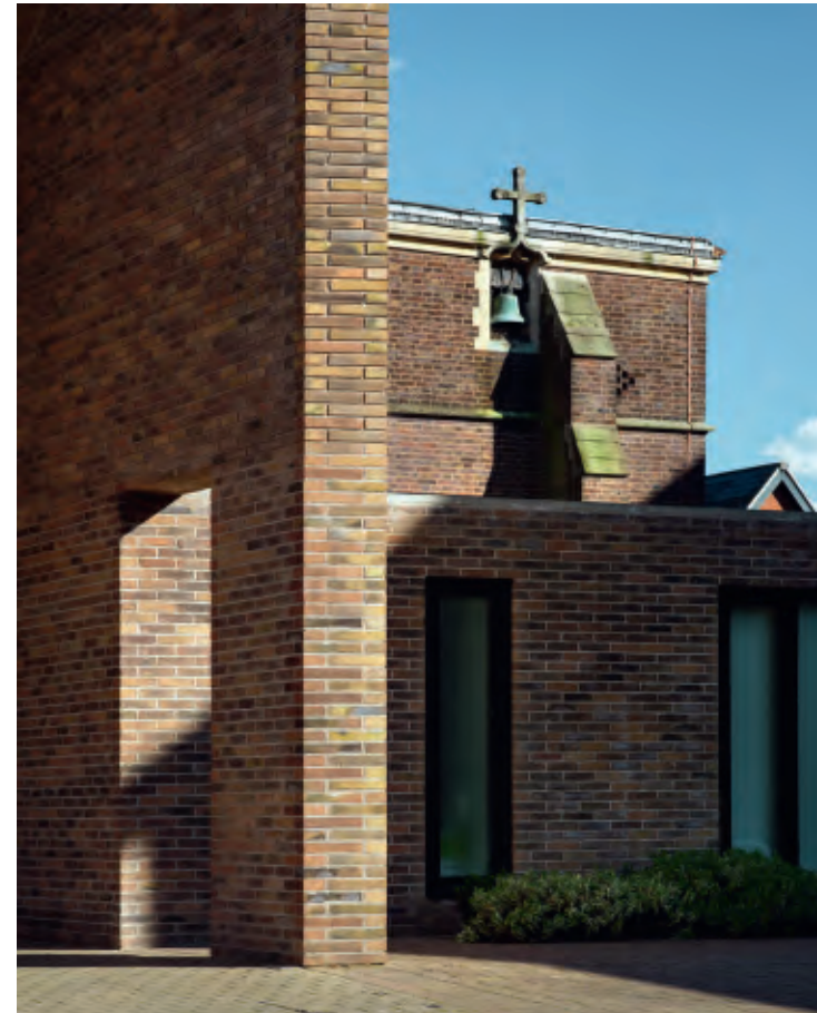
The old chapel's buttresses are just visible in the background, and the new extension fits in nicely with its reddish-brown bricks.
