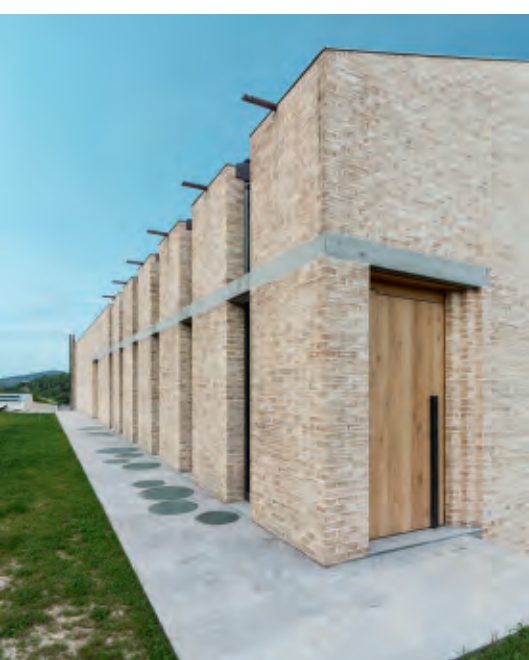
The visible concrete lintels are inspired by 1970s Italian architecture. Circular windows in the paving draw daylight into the basement corridor.
