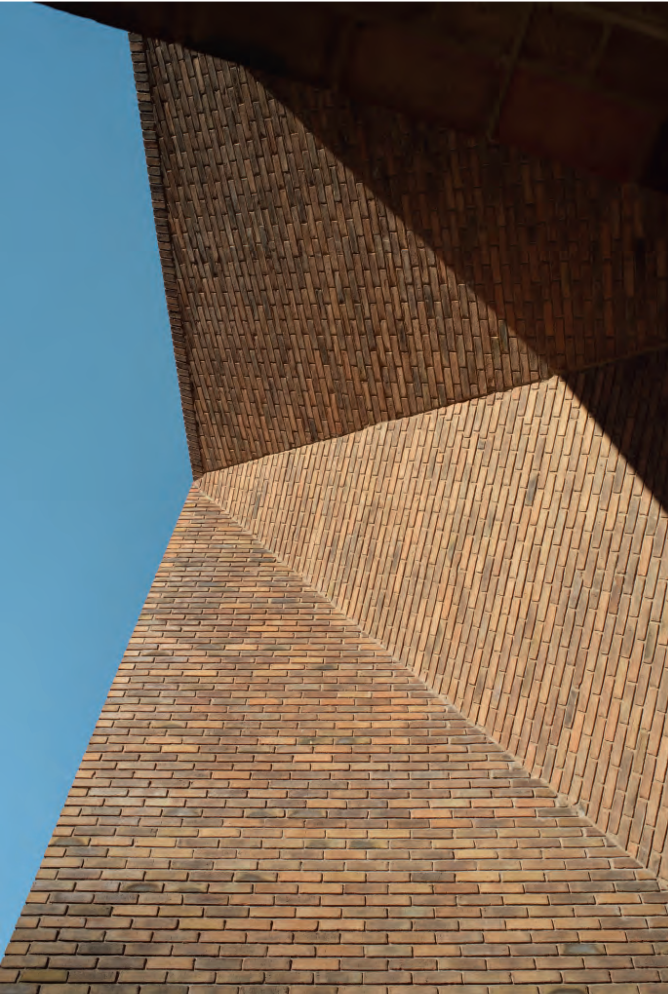
The portal space is clad in the same brick as the rest of the building. Piercy&Company chose the subdued runner bond for all of the brickwork.
