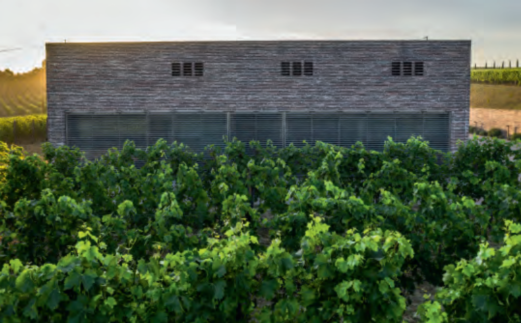
The wooden slats along the east-facing façade provide either partial or complete shade on the terrace.
