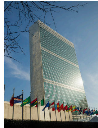
Figure 4.27 United Nations secretariat building: illustrating the east facing glass wall and south stone wall.
