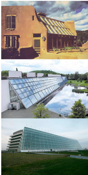
Figure 4.38 Sunspace inspired buildings: (from top to bottom) Balcolm house 1979 - (image credit: Mother Earth News Staff) Science park 1995 - (image credit: Ivy Hughes) Ospedale dell'angelo 2008 -
