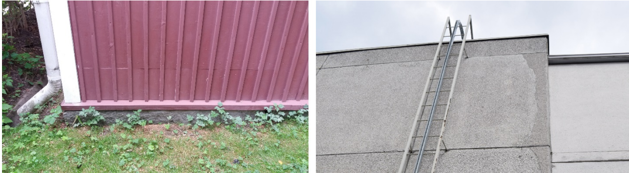
Figure 5. Patch repairs in a traditional wooden building (left) and a modern concrete building (right). Both repairs represent conservation based on the minimal intervention principle, so they also implement CE exemplarily. It is argued, however, that most of the practicing architectural conservationists would find the former acceptable, but fewer would be ready to embrace the latter one.
