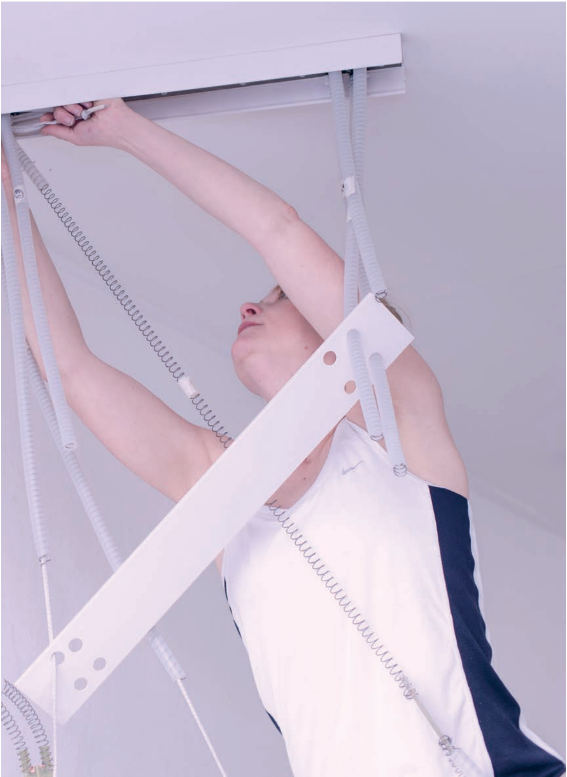
[115] Installation process of the ceiling bars (Image source: Frederik Petersen)
