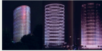
Figure 1-3. Toyo Ito Tower of Winds (1986): From solid appearance, to layered space to transparent skin.
