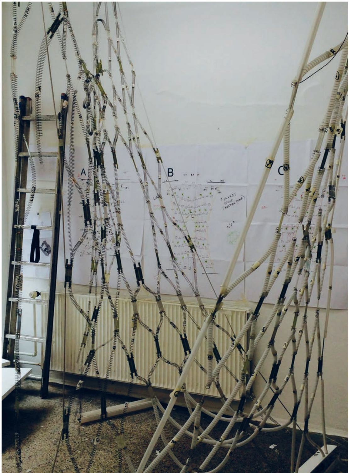
[118] The second layer (middle layer) was added to the first layer
