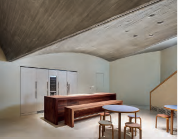
The cellar ceiling is cast in situ and not load-bearing, which meant it could be designed as asymmetric vaults.
