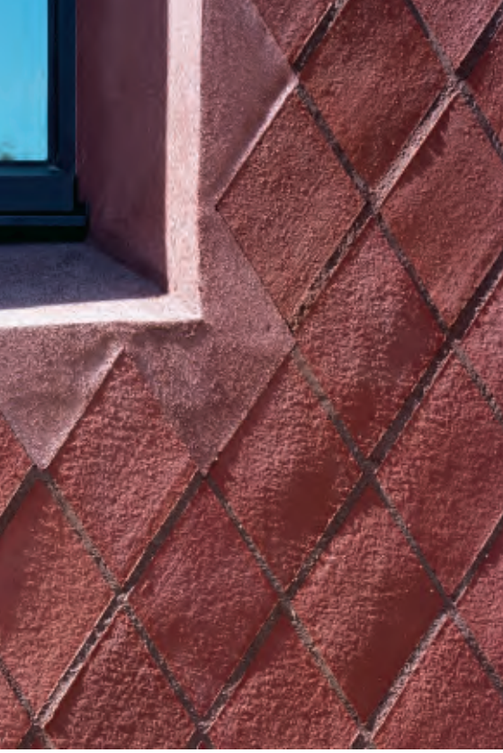
The dimensions of the rhombus-shaped bricks harmonise with the bricks on the neighbouring historic buildings. The handmade bricks' structure responds to the light, bringing the wall to life. Photo: Gion von Albertini
