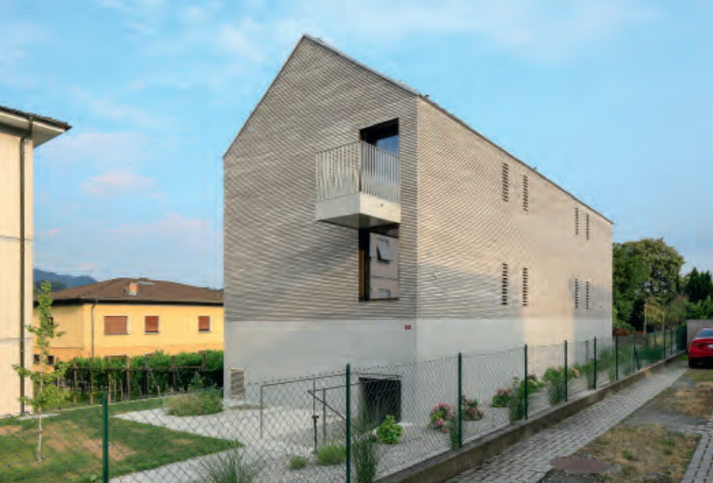
The path to the Atelier runs along the west-facing façade. To ensure privacy in the apartments, the windows on this side have been replaced with interlacing brickwork through which daylight is filtered.
