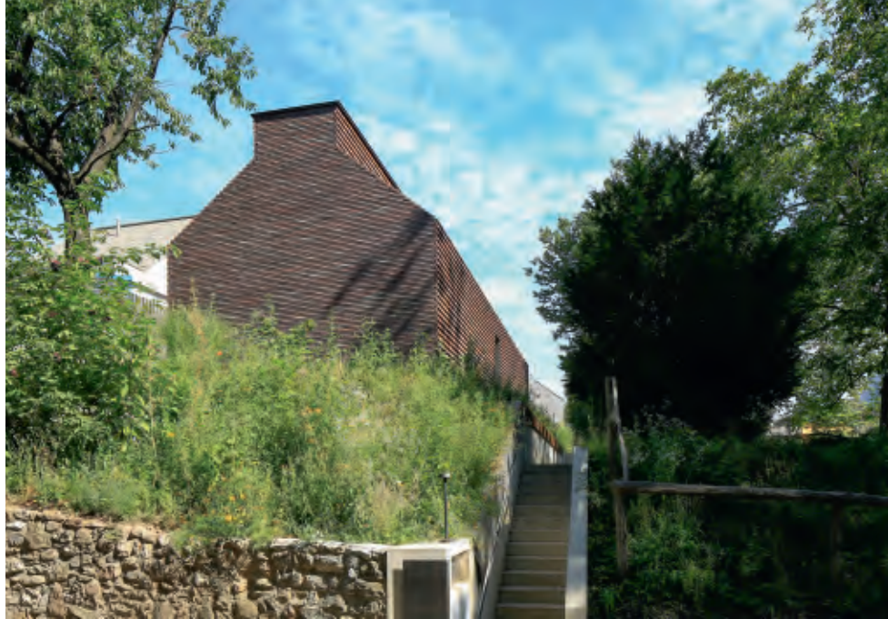
A flight of steps made of in situ-cast concrete leads up to the Atelier from the small forest path. With the red-brown brick façade, the architects sought a quiet contrast to the green surroundings.
