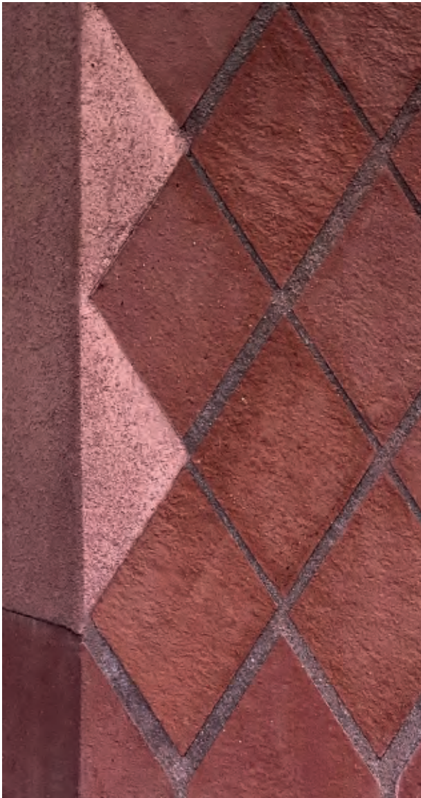
The rhombus-shaped bricks are 37 cm tall, 13 cm broad and 3.7 cm thick. They are laid in 3 mm pre-dyed cement lime mortar, endowing the brickwork with a harmonious sense of wholeness. Photo: Francesca Torzo
