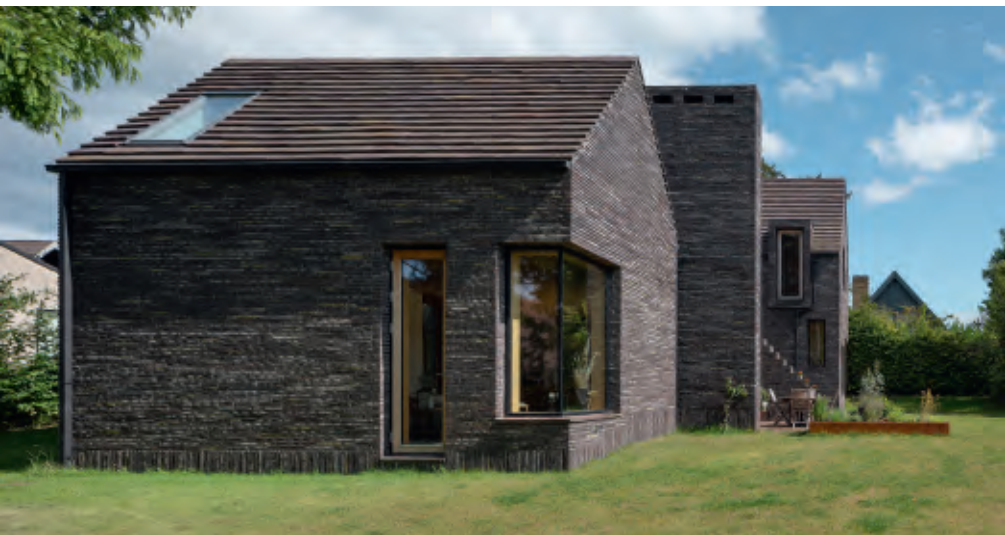
The bricks on the façade and roof are fired from the same type of clay and, along with the precise and tight lines, create a modern, monolithic look.
