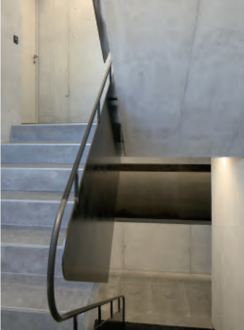
The stairs are made of concrete, with handrails and partial protective screens in an untreated iron finish that patinates, so the black base colour shimmers in green and blue.
