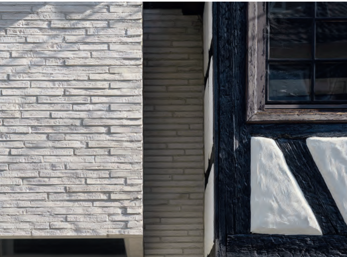
The new extension is clearly differentiated from the building next door, which predates it by more than 300 years, in that its façade bricks are exposed instead of plastered. At the same time, there are similarities between the two in terms of the bright materials and the structure of the plastered surfaces and the hand-moulded brick.
