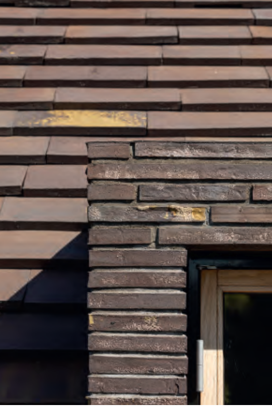
The dormer windows on the roof are framed in Kolumba.
