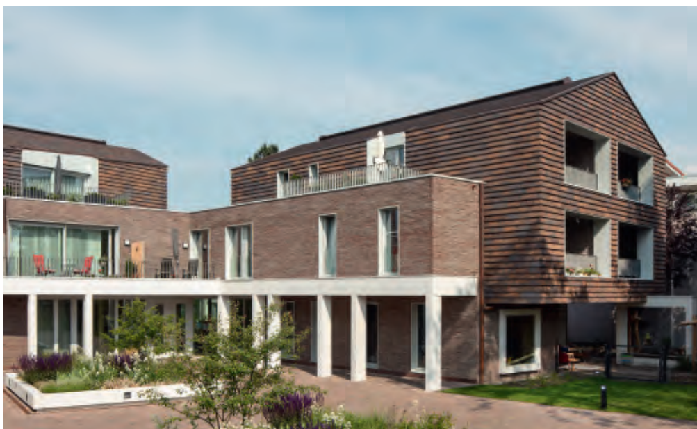
The various parts of the complex are connected only at the ground level. Moving upwards, the wings are configured as three separate volumes, each with its own pitched roof.
