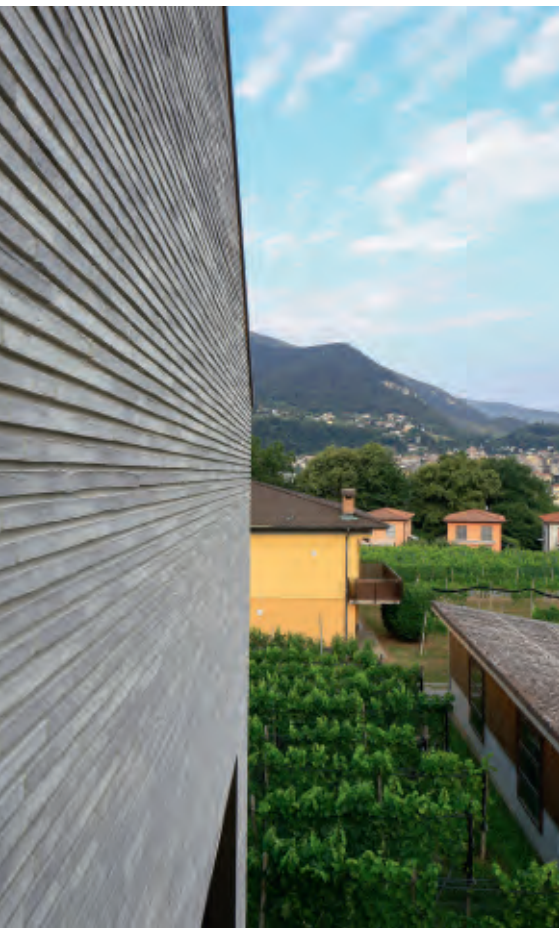
Delicate pale brickwork with recessed bed joints creates a subtle shadow play that, together with the Kolumba, underlines the elongated nature of the building.
