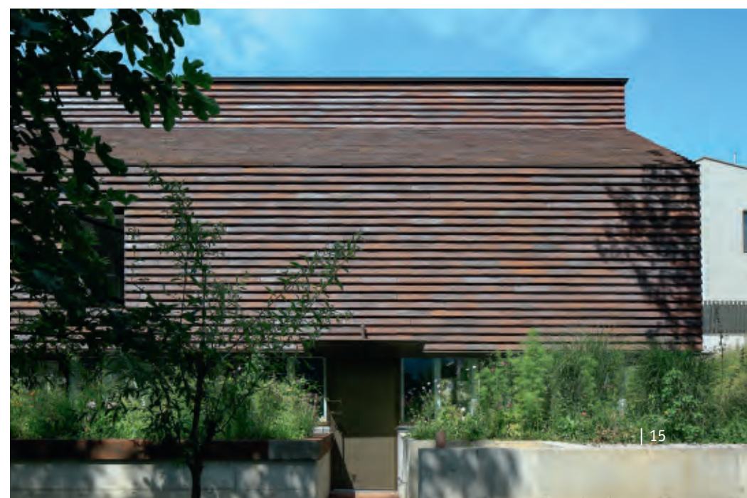
The glass band on the lower façade is slightly recessed from the mass of the brick monolith above, which thus seems to quiver in the air above a green, herbaceous cloud.
