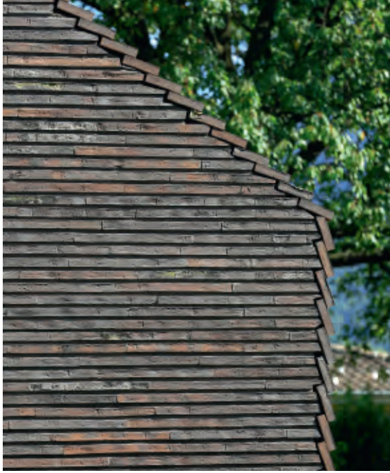
The Kolumba gables have been carefully cut in such a way as to interlock with the bricks on the roof and façade. The result is both minimal and highly detailed.
