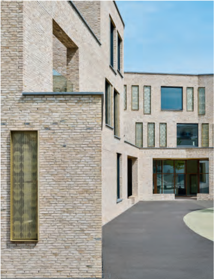
The light bricks relate to the hues of the neighbouring buildings. The grey joints lie flush with the bricks, creating a coherent surface.
