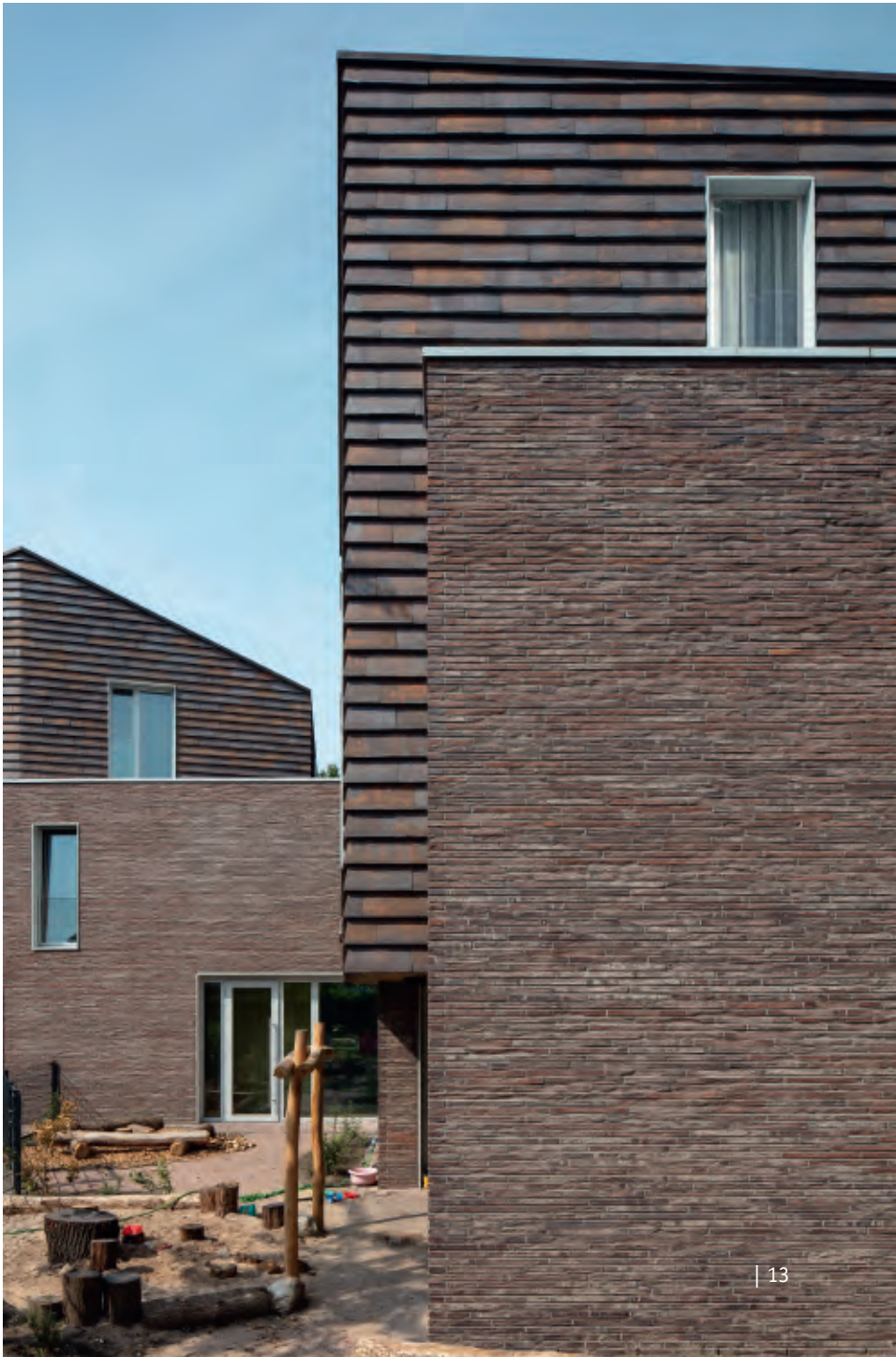
The use of Kolumba and Cover in the same shades of reddish-brown binds together the buildings, while the two bricks' different textures create fine contrasts on the façade.
