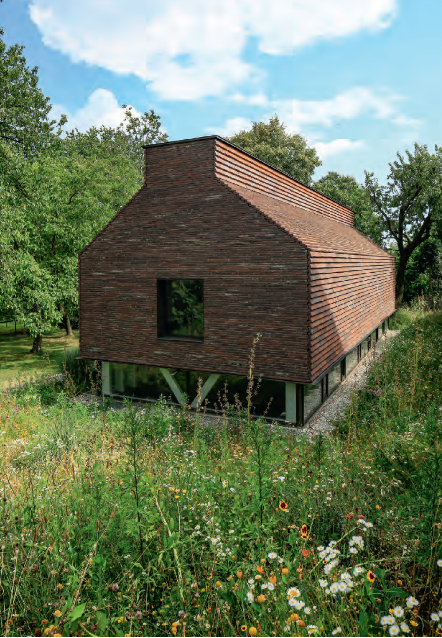
The upper edge of the concrete plinth is on exactly the same level as the terrain. The meeting between residence and garden is mediated by a sharply defined channel, laid in bright, round, polished pebbles, which provides drainage.
