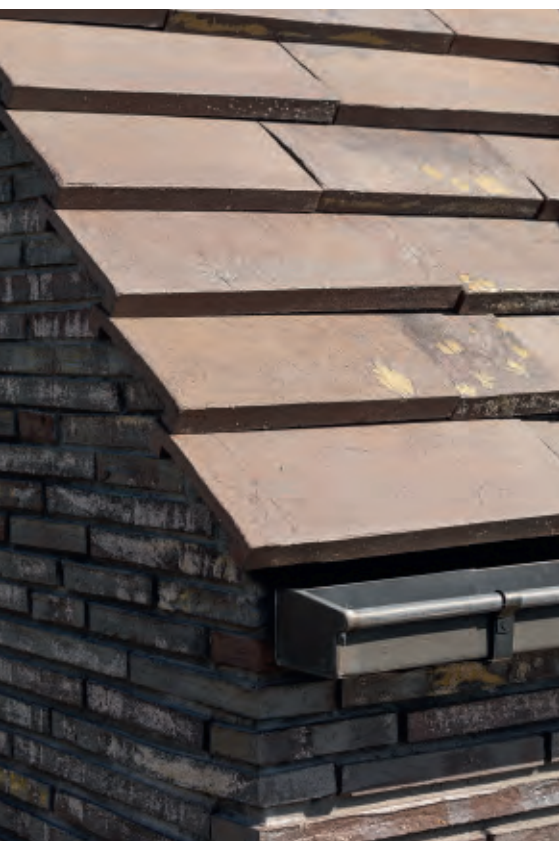
The roof is clad in Cover, fired from the same English clay as the bricks on the façade.
