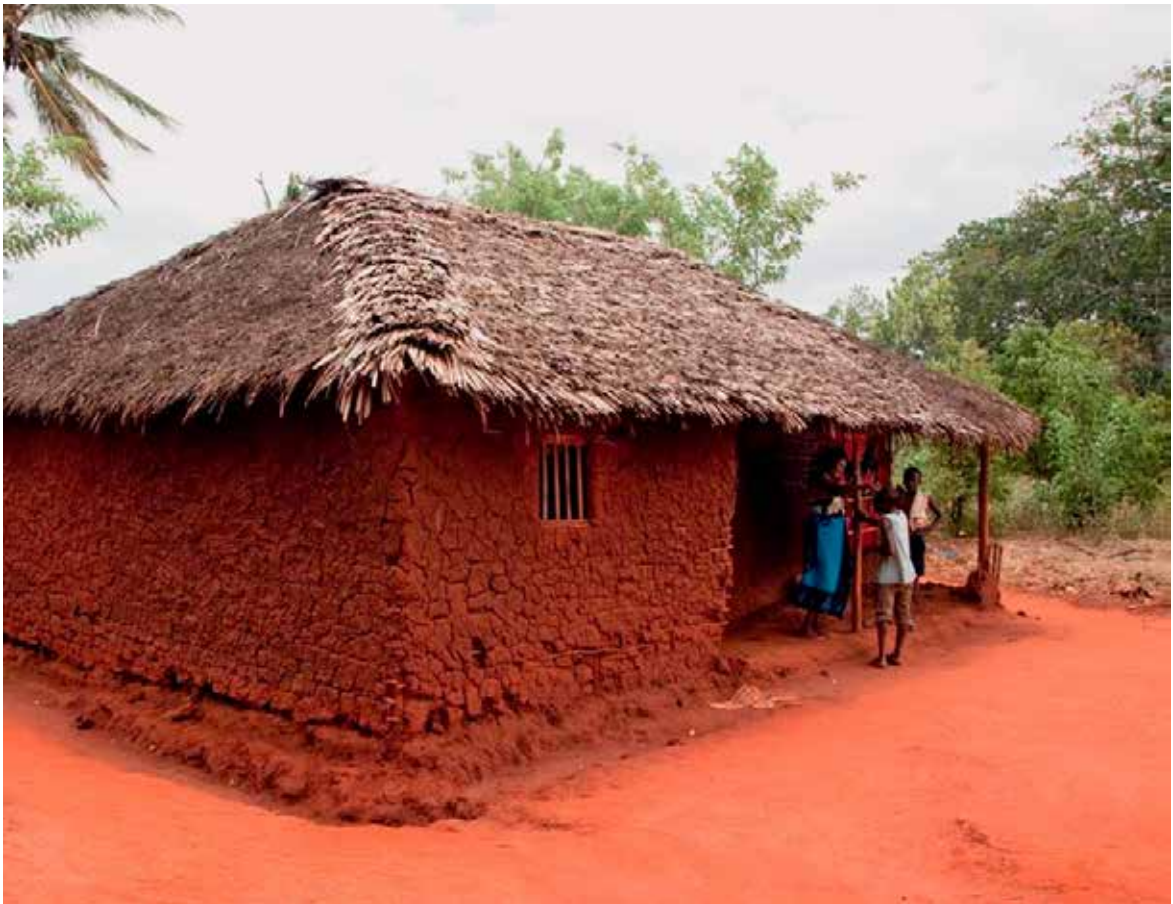
Figure 1: Typical traditional rural house in Magoda, Tanzania: a wattle and daub construction or mud house.
