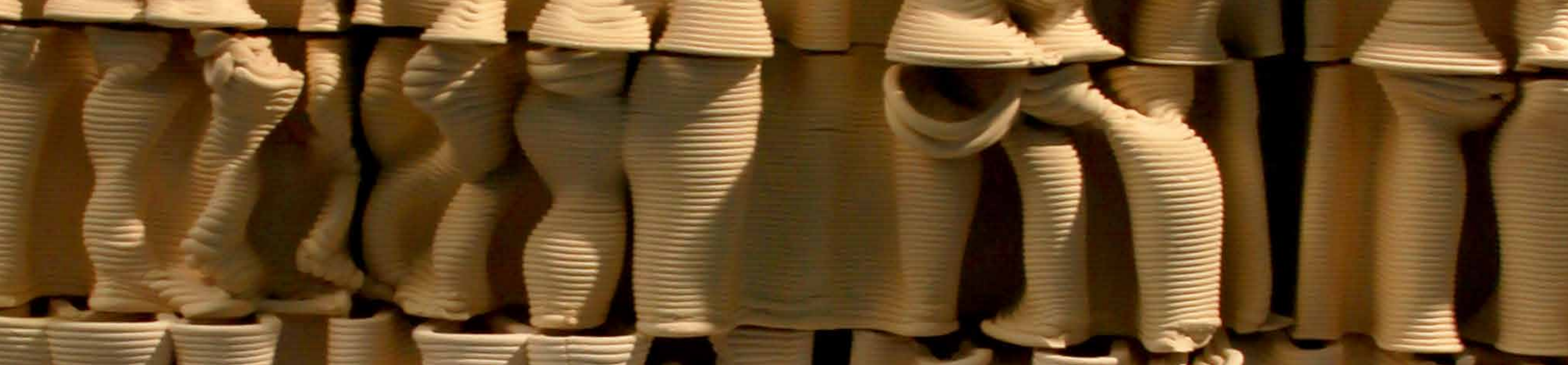
Image Detail of 3D printed ceramic brick wall continued
