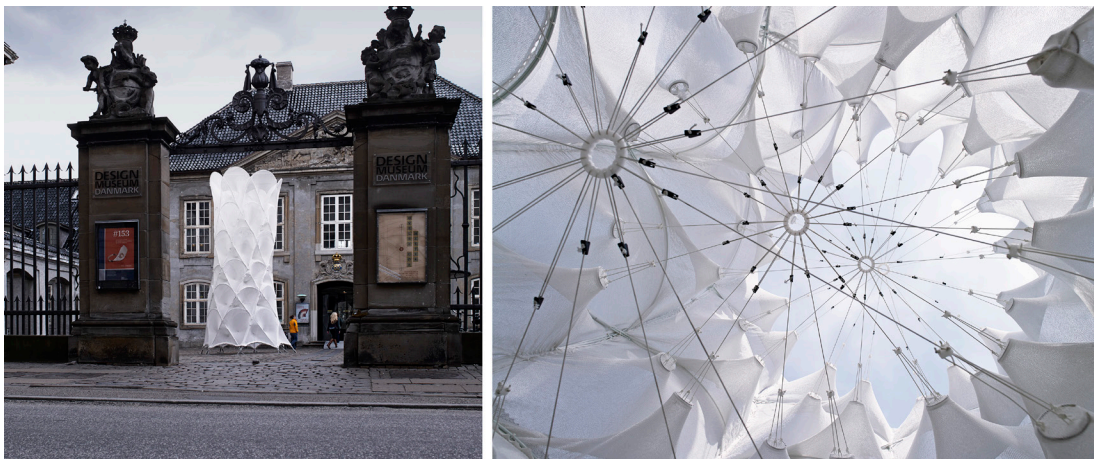
Figure 1: The Tower in the Courtyard of the Danish Design Museum. The interior of the Tower is characterised by the tensioning system and the resulting cone-like membranes. Photo: Anders Ingvarsen.:
