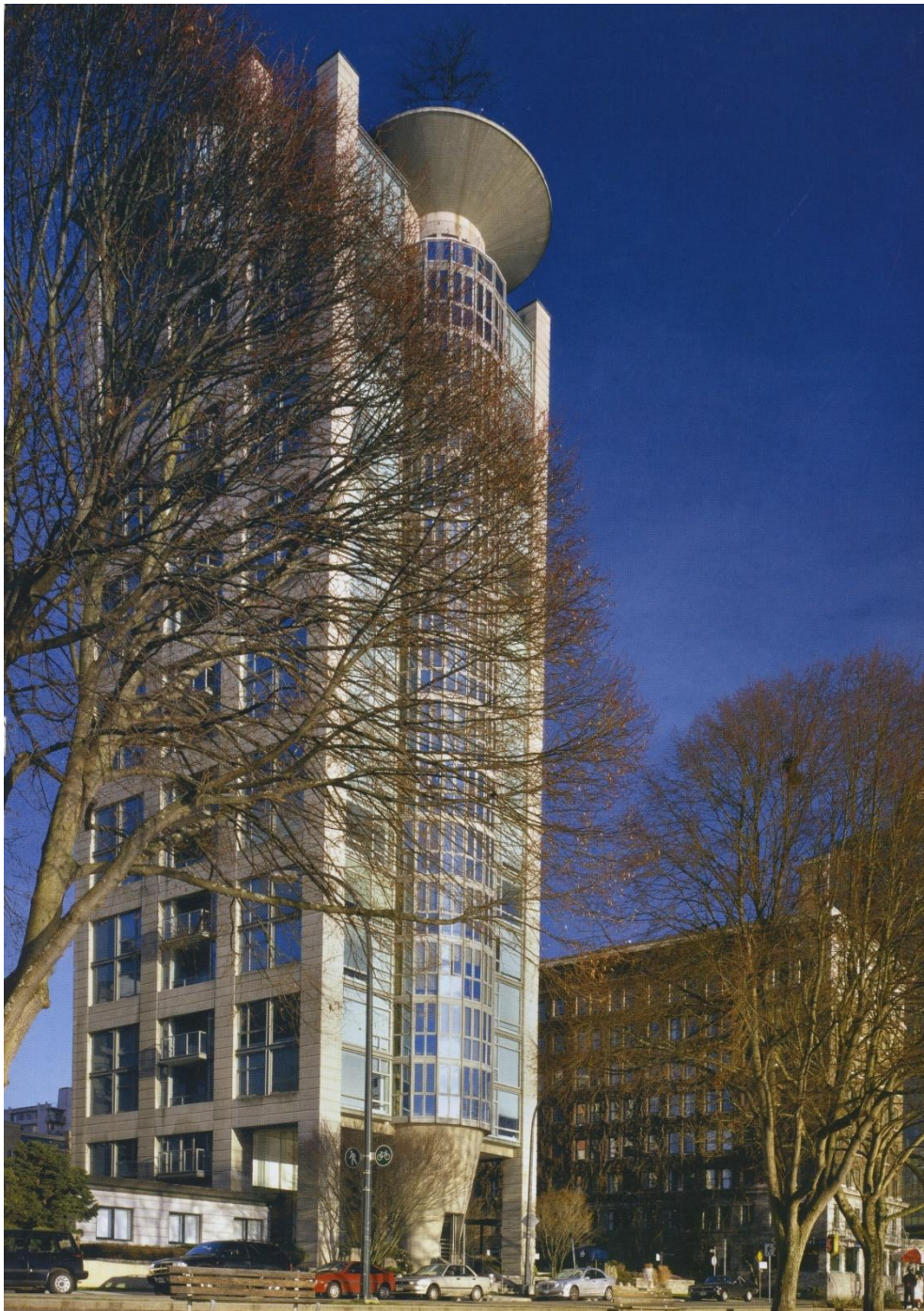
Fig. 39 Richard Henriquez: Eugenia Place Tower , West End Vancouver Photograph of Southwest Facade
