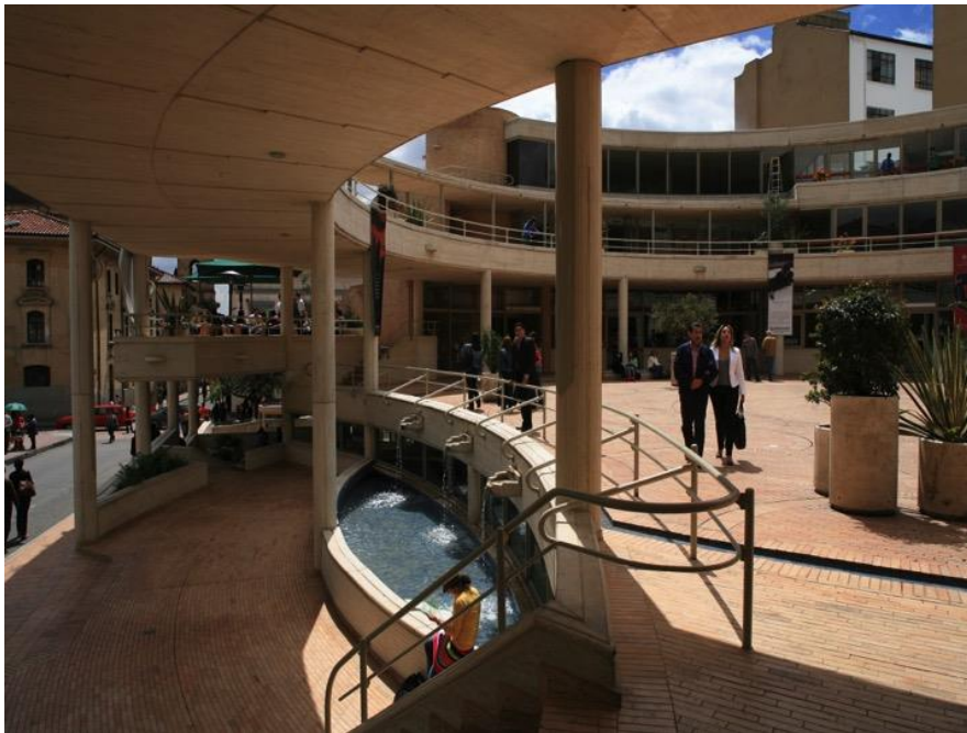
Fig. 3: Closure and support elements in the Garcia Marquez Cultural Center. Picture: Carolina Cantor.
