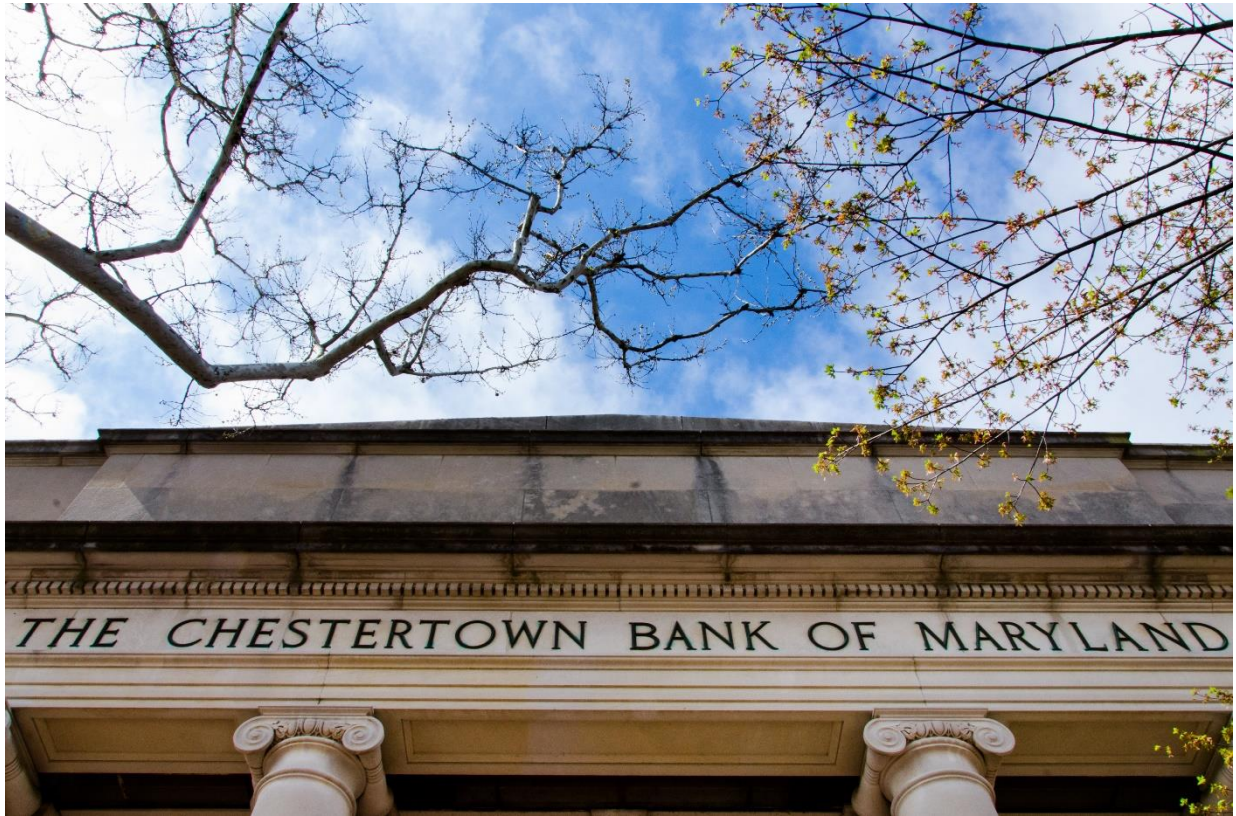
Fig. 5: Chestertown Bank façade. (Photo: Zachary Z. Handler)
