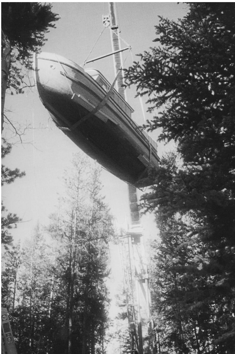
Fig. 13 Richard Henriquez, Leighton Studio , Banff Construction Photograph
