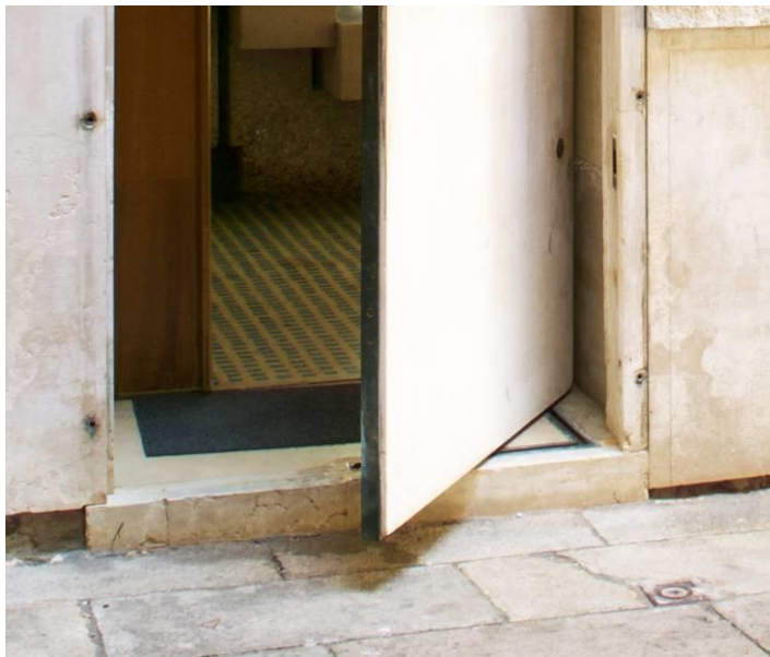
Fig. 21: Olivetti Showroom Floor Detail.
