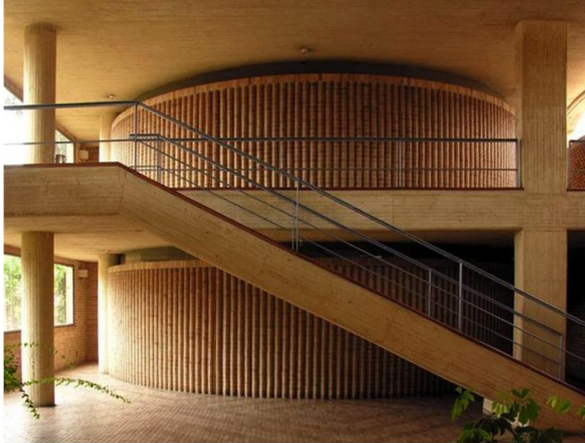
Fig. 4: Contrast between brickwork and concrete, between closure and support elements. Picture: Carolina Cantor.
