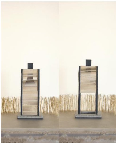
Image 17: Operable screens provide protection from the wind or open to a view. When not in use, the screens on all four sides are closed.
