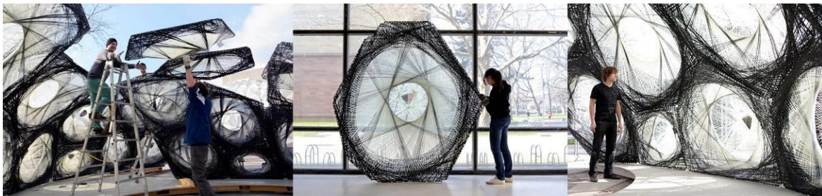
Pict 6: ICD/ITKE Research Pavilion 2013-14 in progress by students
