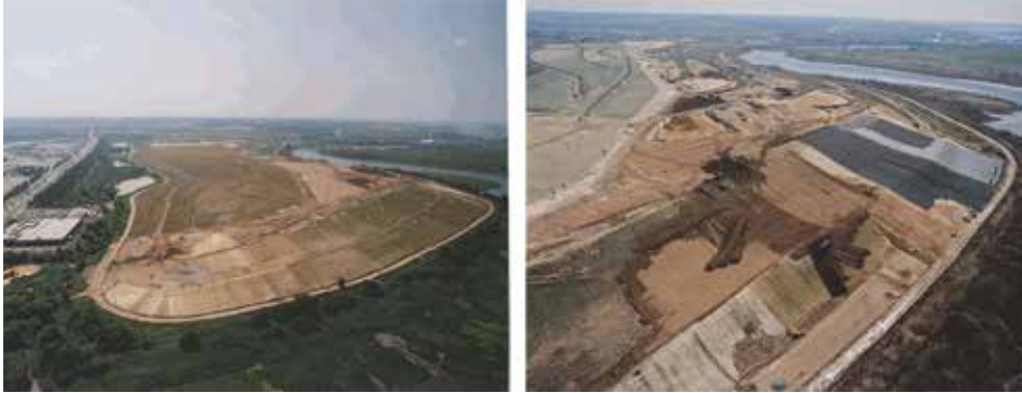
Figure 7: (Photos kindly deposited by Tully Construction Co., Inc.) The installation of 'final cover' (also called the landfill cap) on Fresh Kills Landfill. The final cover is composed of a series of layers of soil, synthetic textile, plastic, and grass and is complemented by construction of adequate and sometimes elaborate drainage systems and basins.
