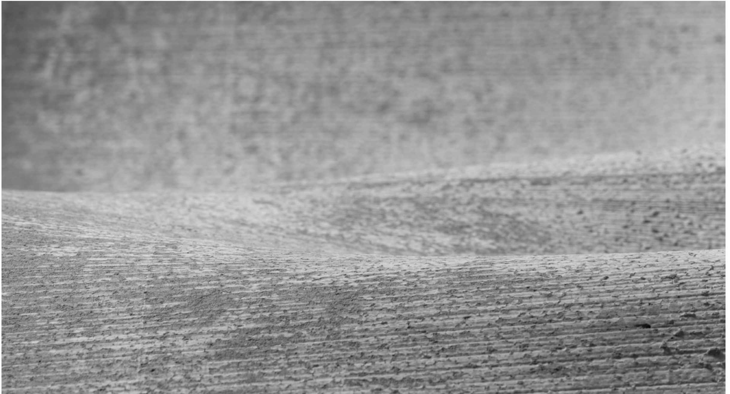
Close-up photo of a concrete surface. The surface is a result of hot wire cutting, EPS material texture, retarder surface treatment, and the concrete casting. All processes are visible in the final result.
