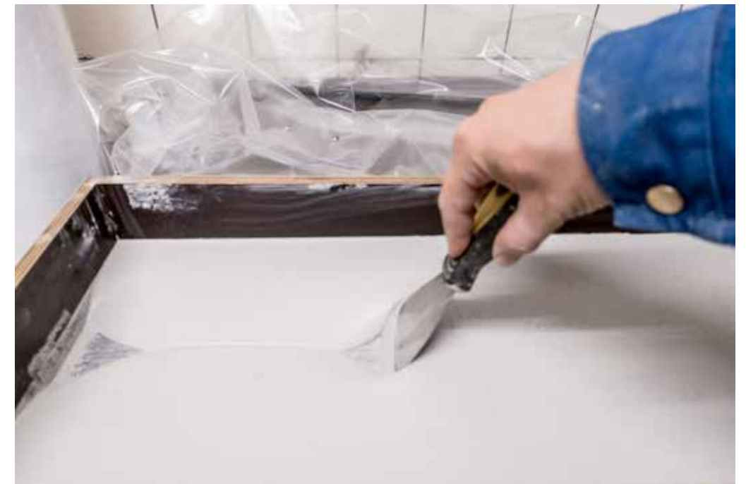
Manual manipulation of fluid concrete. The materiality is captivating. The constantly changing viscosity is also a continuous change of potential form.
