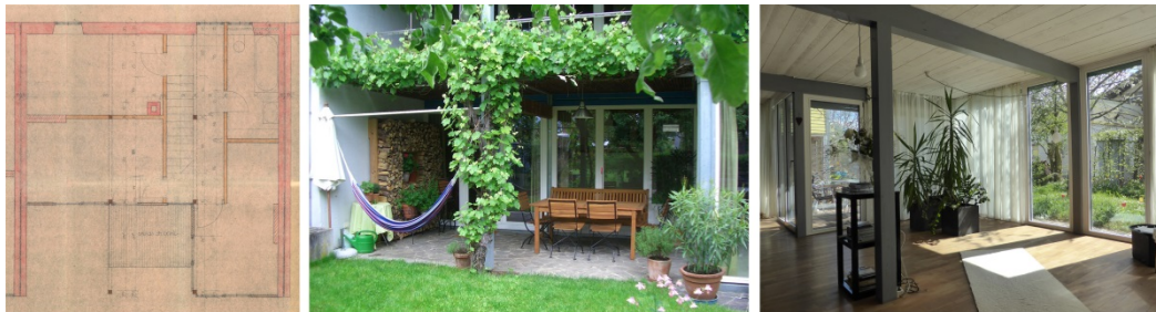
Fig.5 left: hand-drawn plan of upper floor of the smallest unit with loggia, outdoor column and balcony. Red = brick, brown = wood. Centre: loggia of the same house Right: living room with freestanding column in the space and unpolished slab. (pictures taken 2015)
