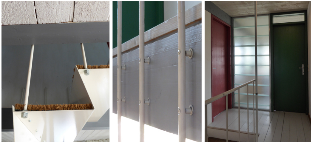
Fig.3 hanging stair of inexpensive and adjustable steel elements, screwed in glulam beams
