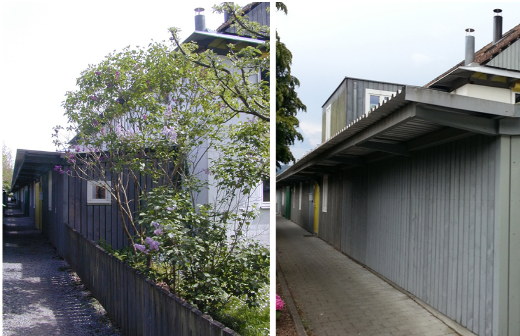
Fig. 6 Northern corridor 1988 and 2000 with vertical extension and transformed fence to wall
