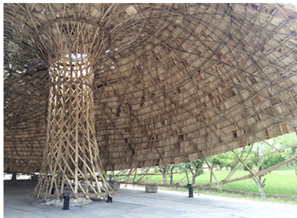
Fig 2: COCOON I. Interior with split bamboo construction
