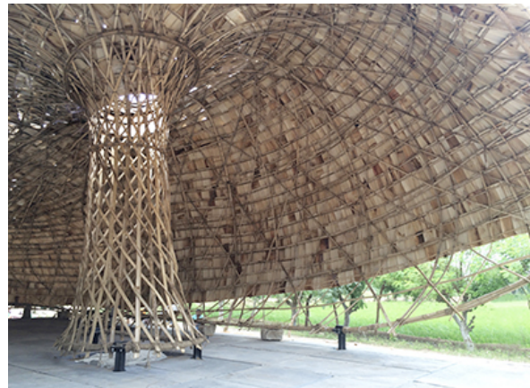
Fig 2: COCOON I. Interior with split bamboo construction
