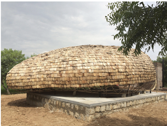
Fig 1: COCOON I. Bamboo building with shingle roof in bark
