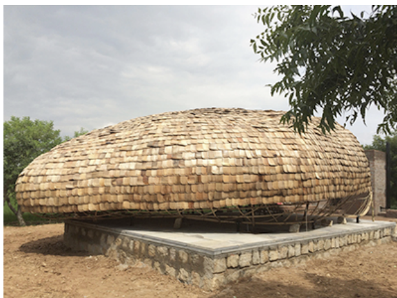
Fig 1: Building part of bamboo and granite with shingle roof in bark. Fig 2: Interior of split bamboo construction and woven column.
