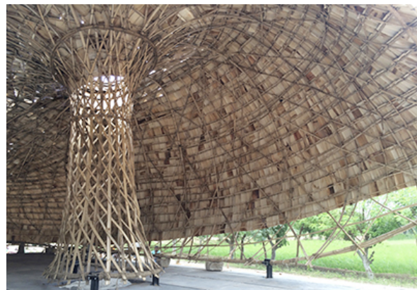
Fig 1: Building part of bamboo and granite with shingle roof in bark. Fig 2: Interior of split bamboo construction and woven column.
