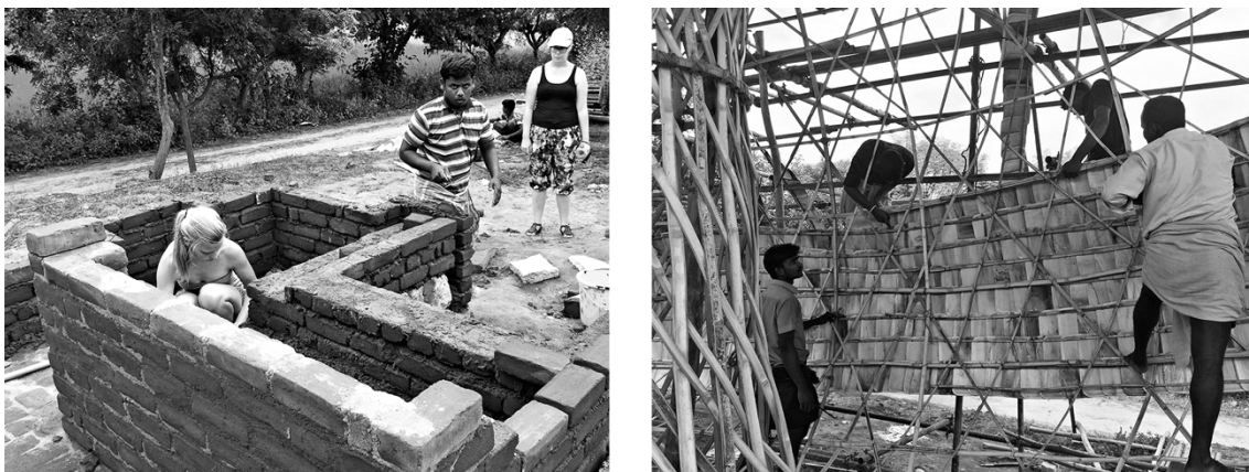
Figure 5. Cross-cultural building process of eco toilet and bamboo construction
