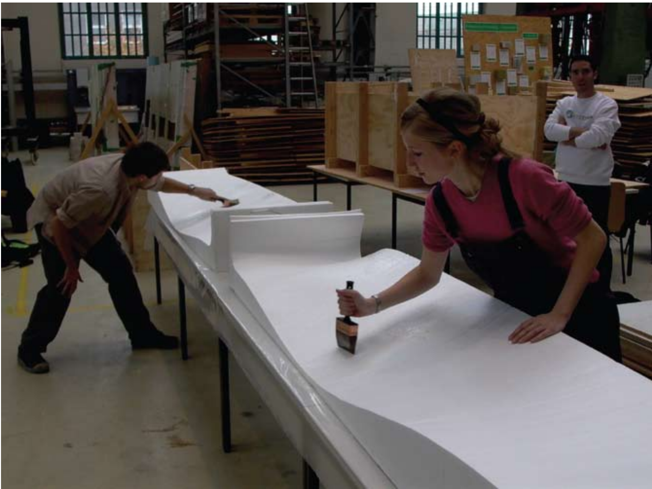
Treating the inside of moulds with a wax-oil solution.
