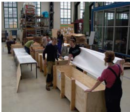
Assembling the formwork. Mounting the inside polystyrene moulds in an outside load bearing structure of plywood and rafters.
