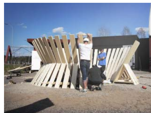
Assembly of the installation
