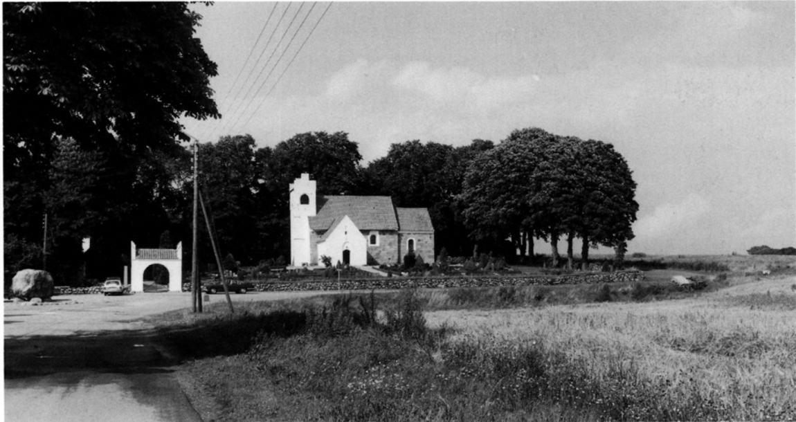
Fig. 1. Kirken set fra syd. NE fot. 1985. - The church seen from the south.
