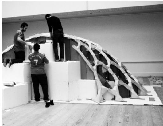
Figure 10: The structure being assembled against the parametrically generated falsework.
