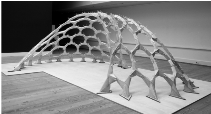
Figure 6: The ReVault case study: A concrete grid shell pavilion made up of 110 discrete elements.
